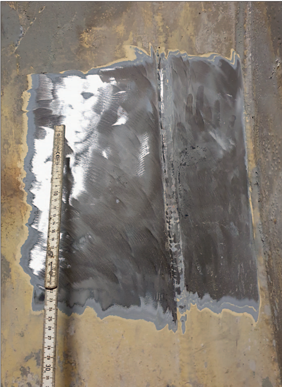
Damaged area prepared for removal.
