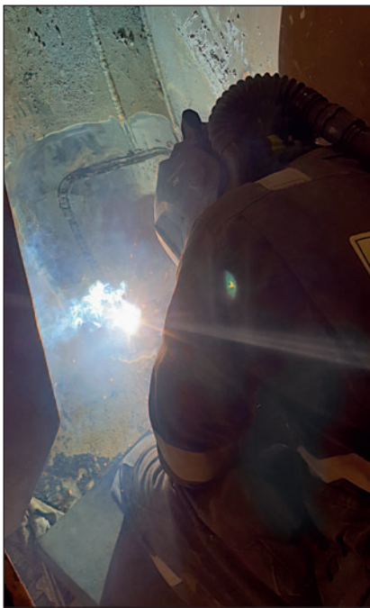
Welding the insert.
