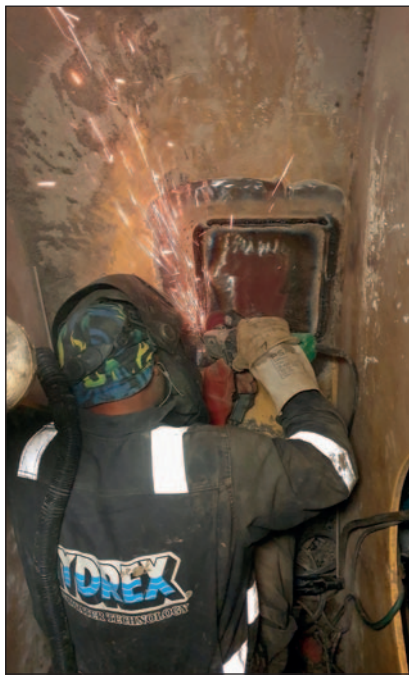
Hydrex diver/technician working on the edges of the insert.
