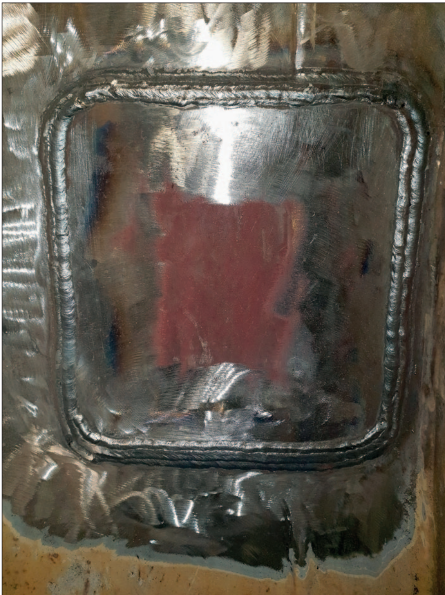
Fully welded insert.
