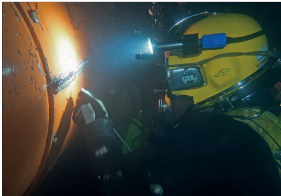
Reinstallation of one of the rope guards.
