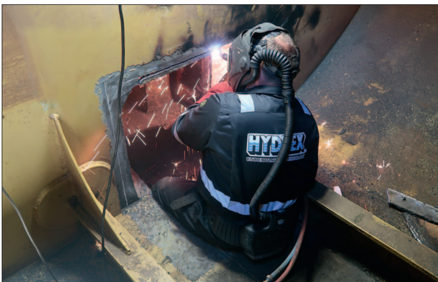
An insert repair on the bulkhead of a vessel that grounded. The repair was rapidly completed without a trip to drydock.
