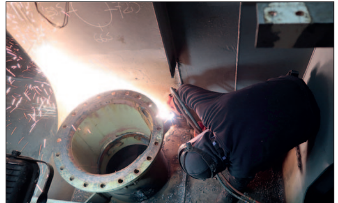
One of our men during emergency scrubber overboard repair in Denmark.
