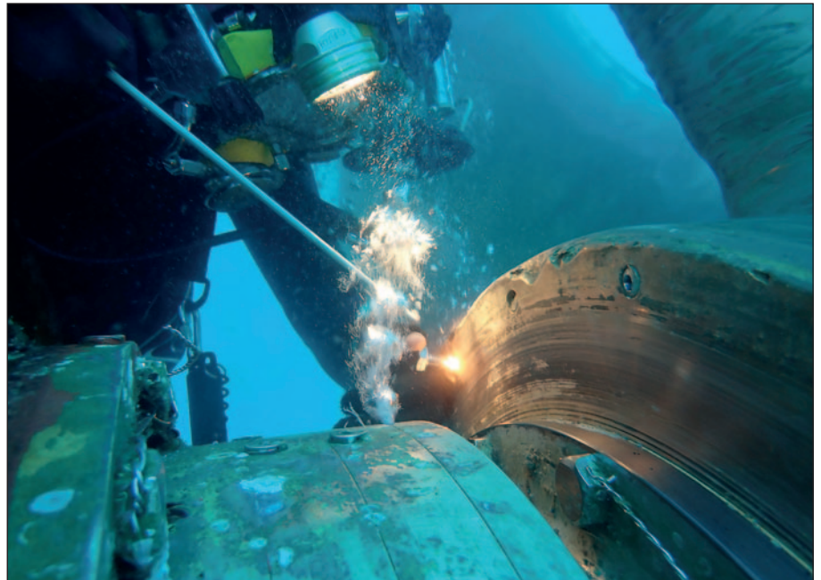
Welding new studs on the broken bolts that could not be removed.
