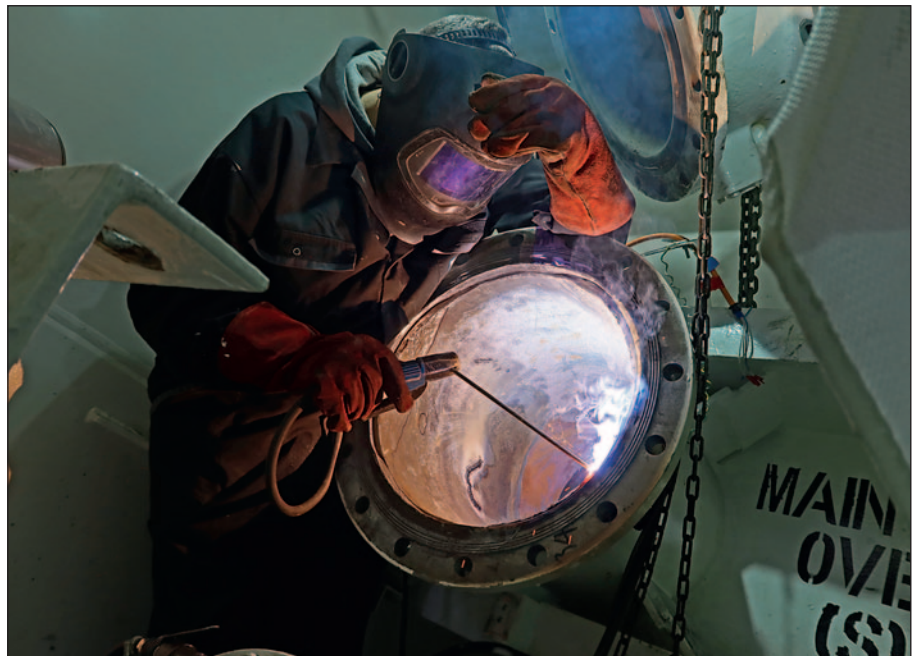
Hydrex welder during scrubber pipe repair.
