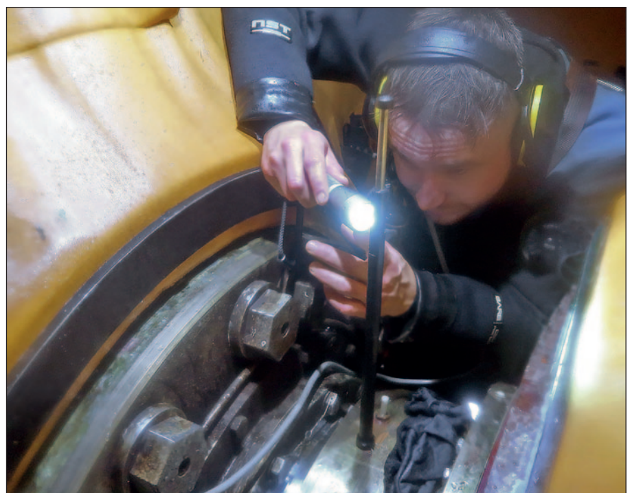
Hydrex diver/technician taking shaft wear down reading.
