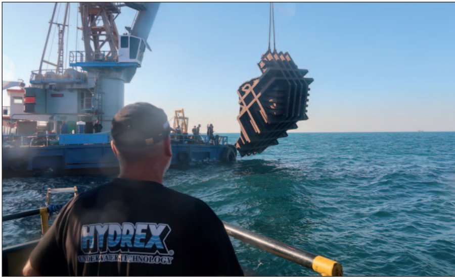
Crane barge moving the cofferdam into position.
