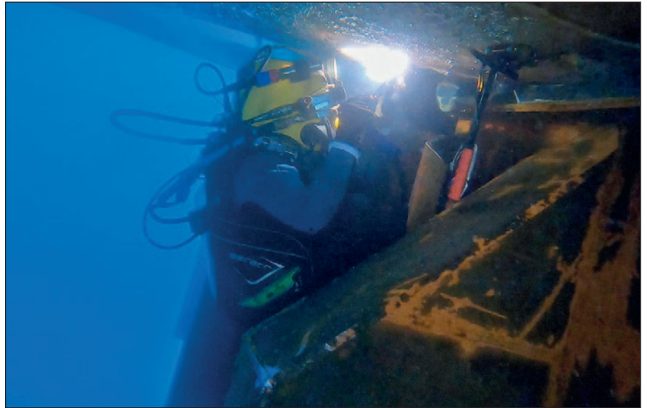
Welding the cofferdam in place.
