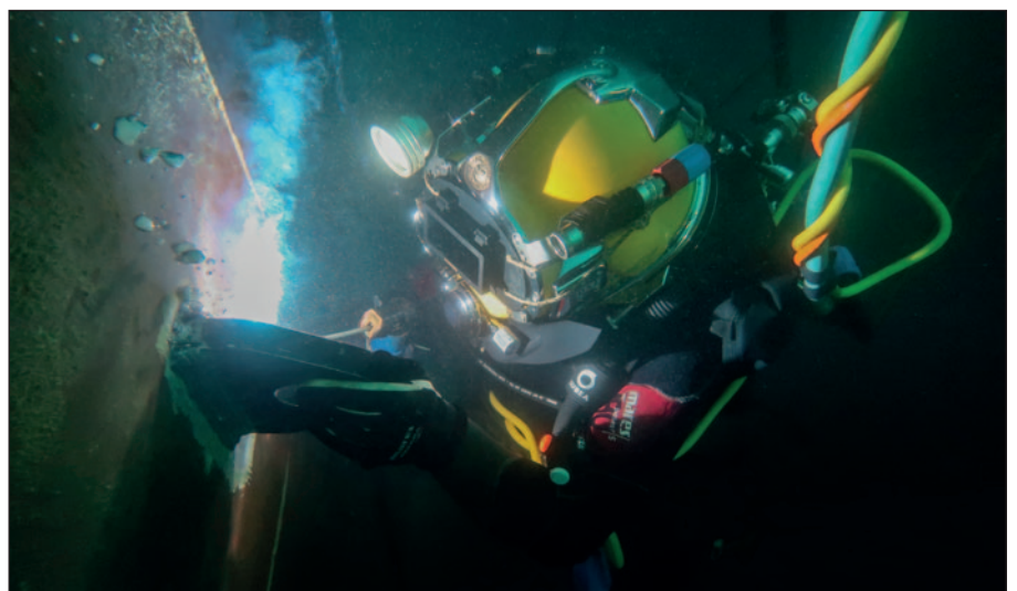
Welding padeyes on the hull.
