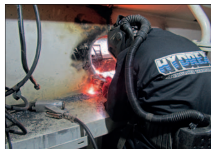
Scrubber pipes repaired and given lasting protection 11-14
