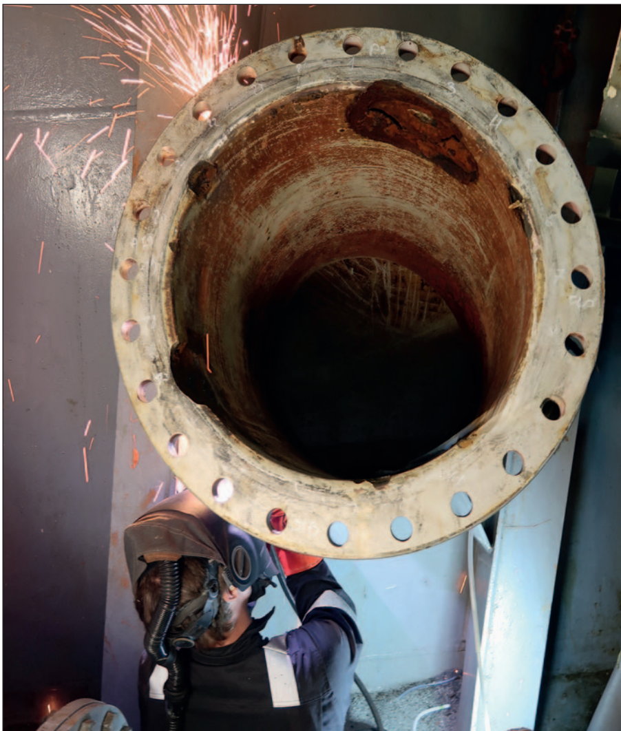
Removing the old scrubber pipe.
