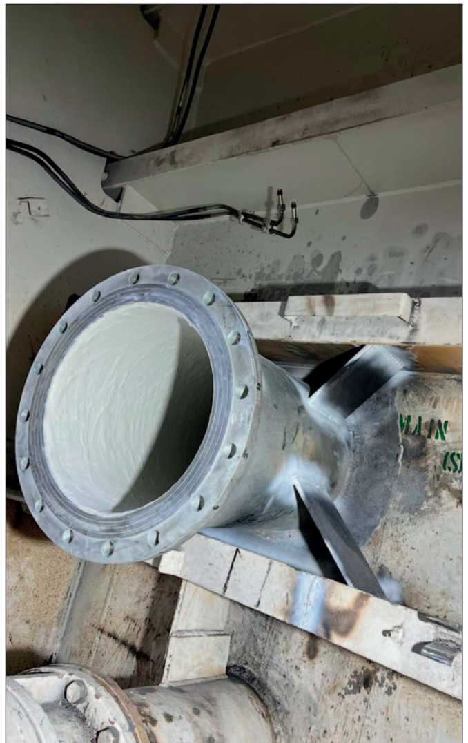
New scrubber pipe. The inside was coated with Ecospeed.
