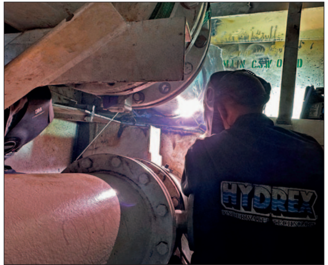
Hydrex diver/welder during installation of a new scrubber pipe.
