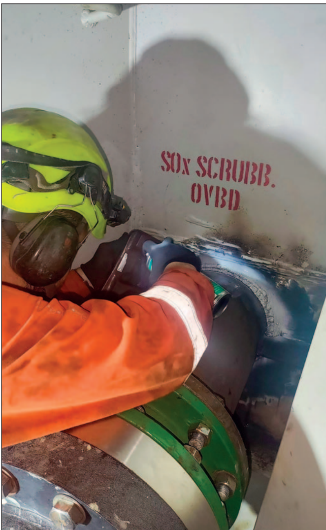
Independent inspector checking the welds.
