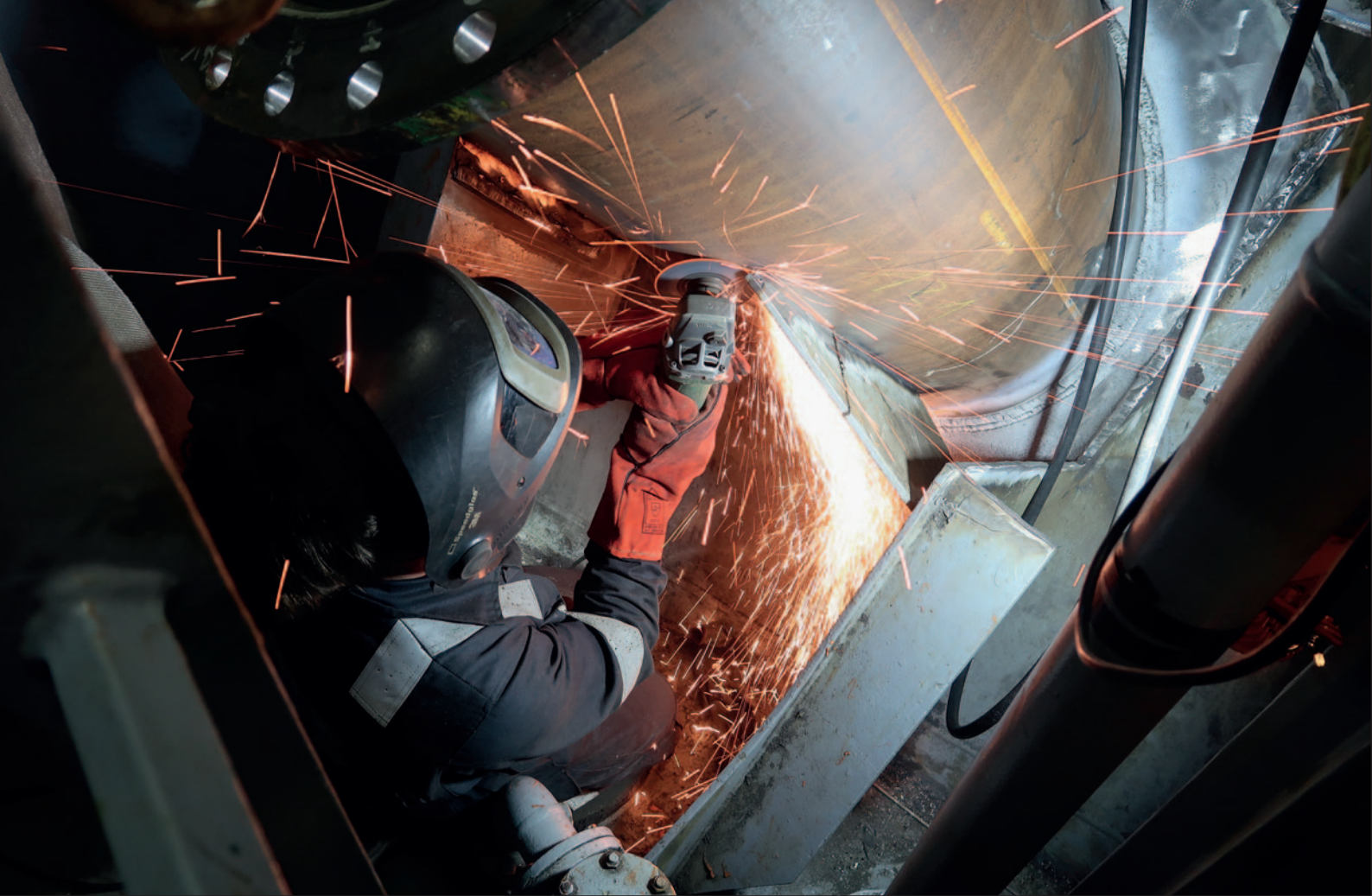
Cutting away the brackets of the old pipe.
