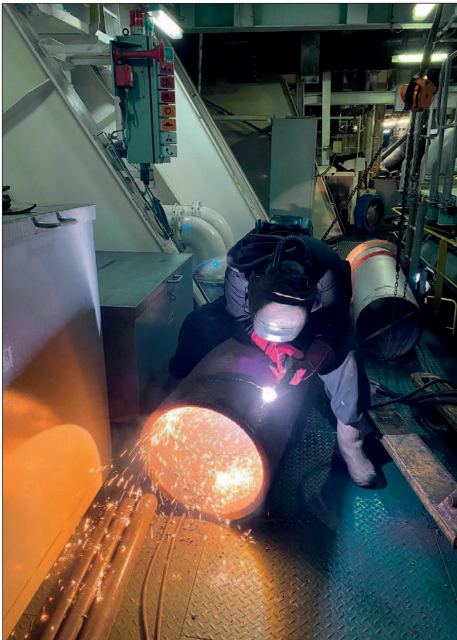
Preparing the new scrubber pipe for installation.
