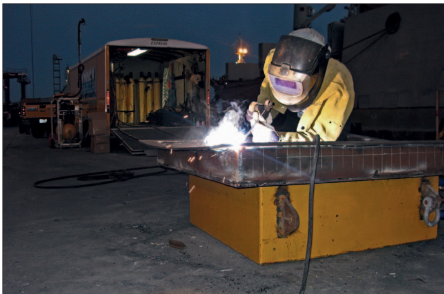
Preparing the cofferdam for installation on ro-ro vessel.
