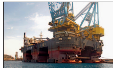
Underwater removal and reinstallation of 60-ton azimuth thruster in Cartagena 10-11
