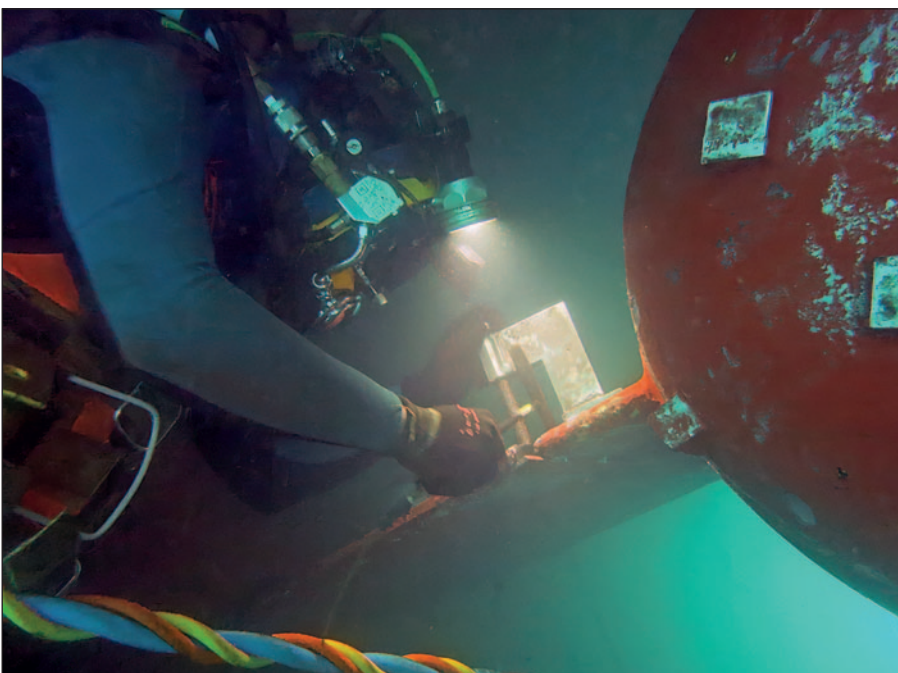
Preparing the old bow thruster for removal.
