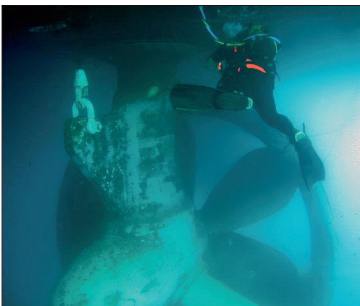
Hydrex diver/technician guiding azimuth thruster during removal.
