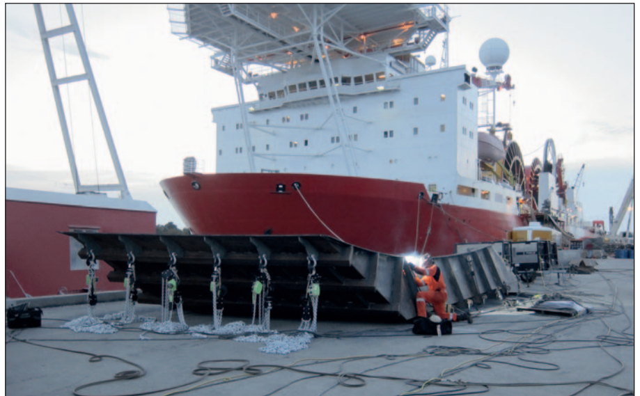
Final touches being made to one of the open top cofferdams.
