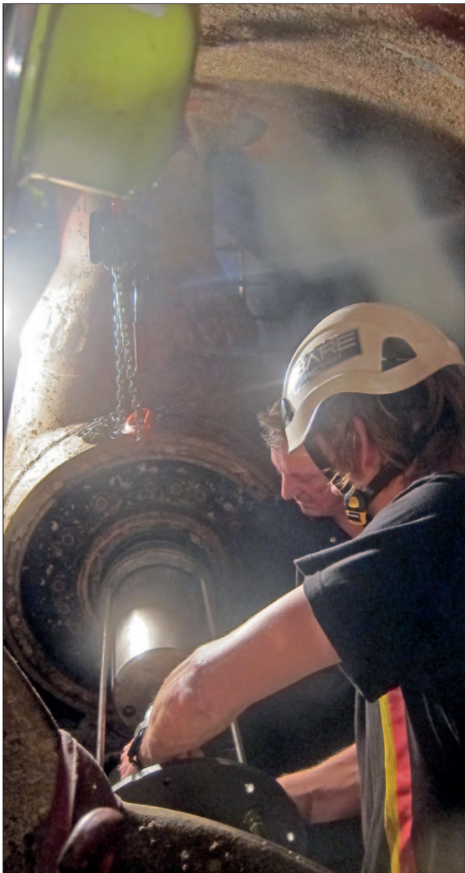
Pulling the liner out of the bow thruster unit.
