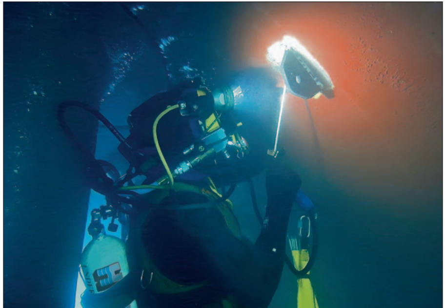
Hydrex diver preparing the thruster tunnel for removal of the unit.
