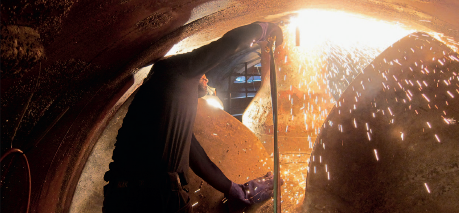
Hydrex technician working on the rigging points in the thruster tunnel.
