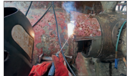
Underwater thruster repairs 4-5
