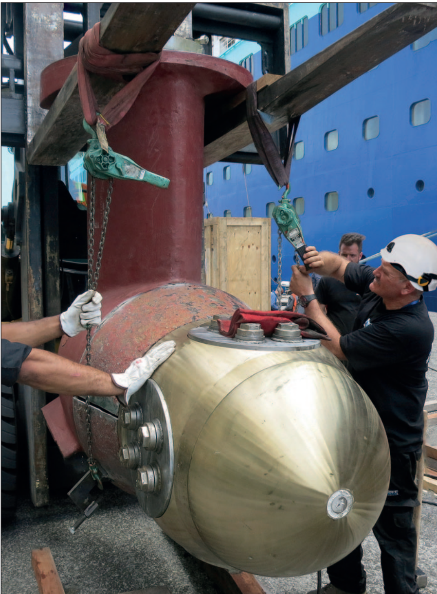
Preparing the new unit for installation.
