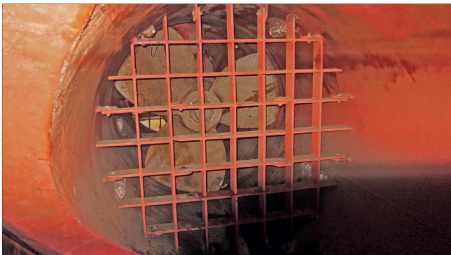
Bow thruster tunnel ready to be flooded again after the repair.
