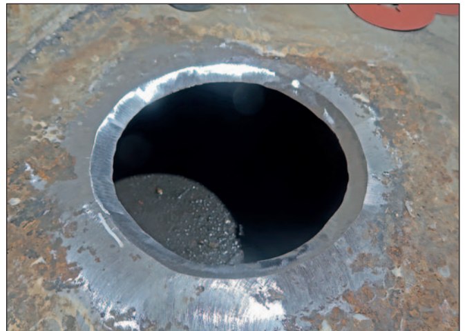
The damaged area was removed and the edge of the hole was prepared for installation of the new insert.
