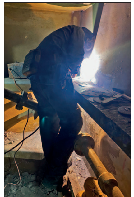
One of our welders during crack repair in Zeebrugge.
