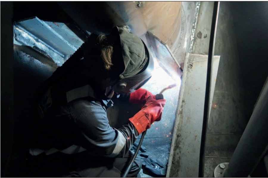
The frame and brackets are cut through to make way for the new pipe.
