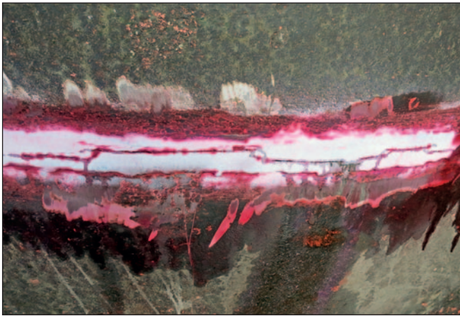
A dye check revealed the extent of the cracks.
