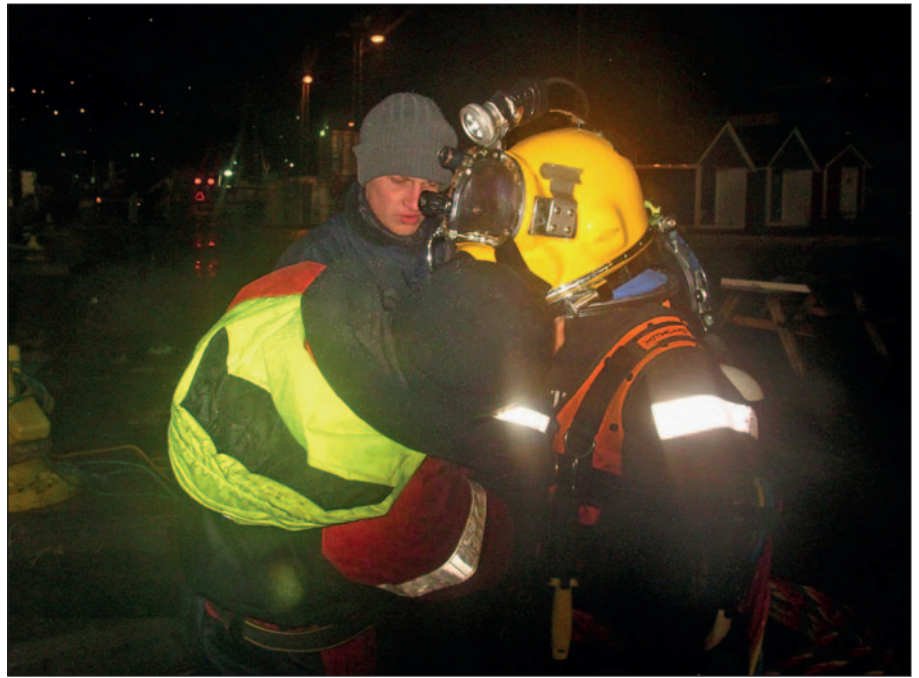
Hydrex diver getting ready for underwater repair.
