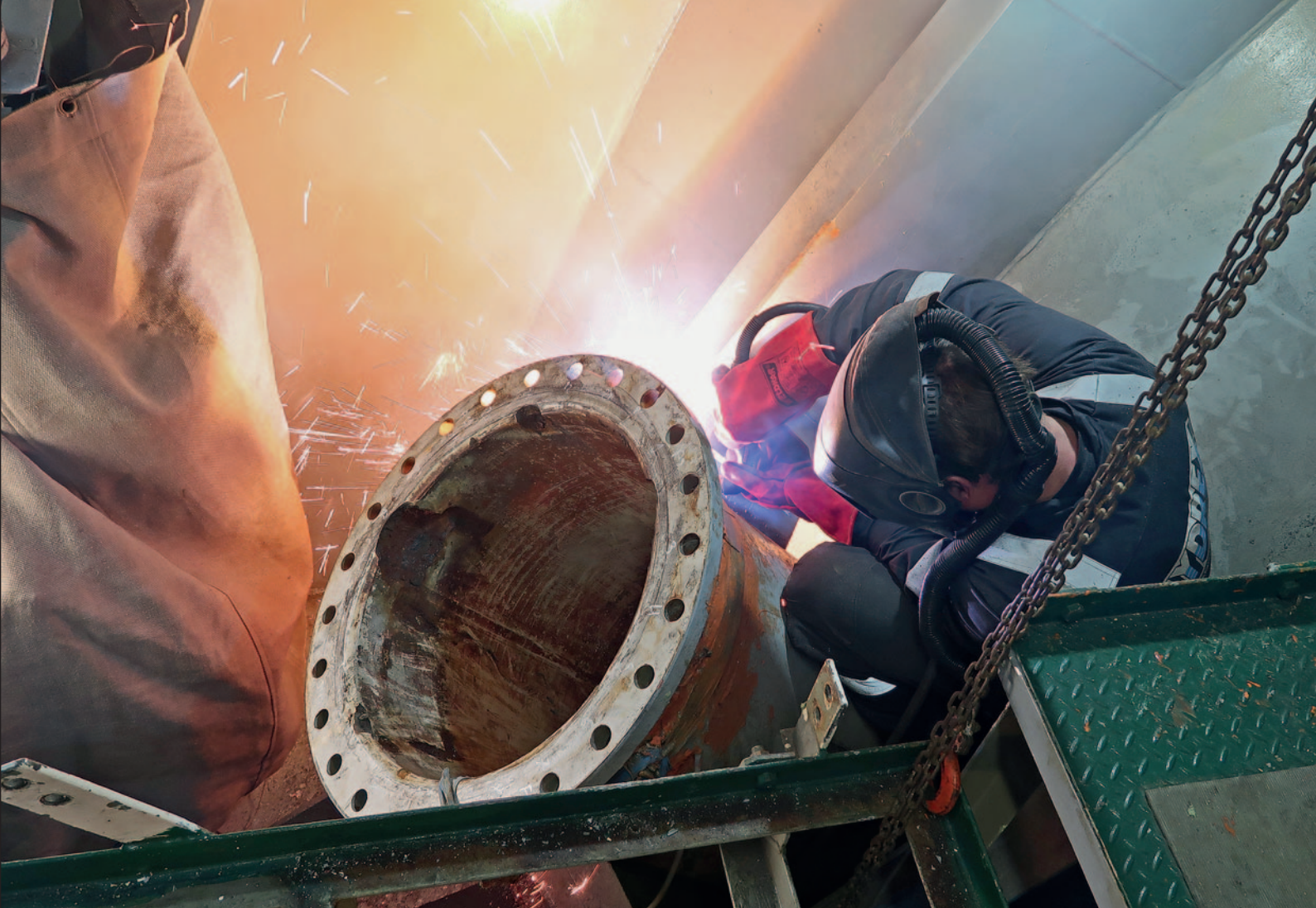
Hydrex technician cutting away the old pipe.
