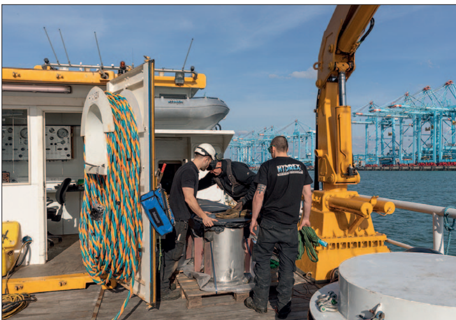
Preparation on board one of our workboats for a scrubber pipe operation.
