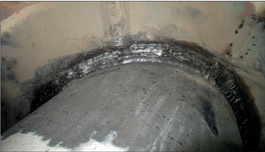
New scrubber pipe after welding.
