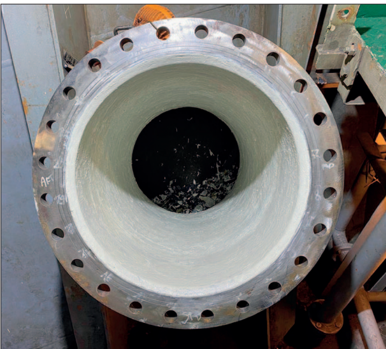
New scrubber pipe coated with Ecospeed.
