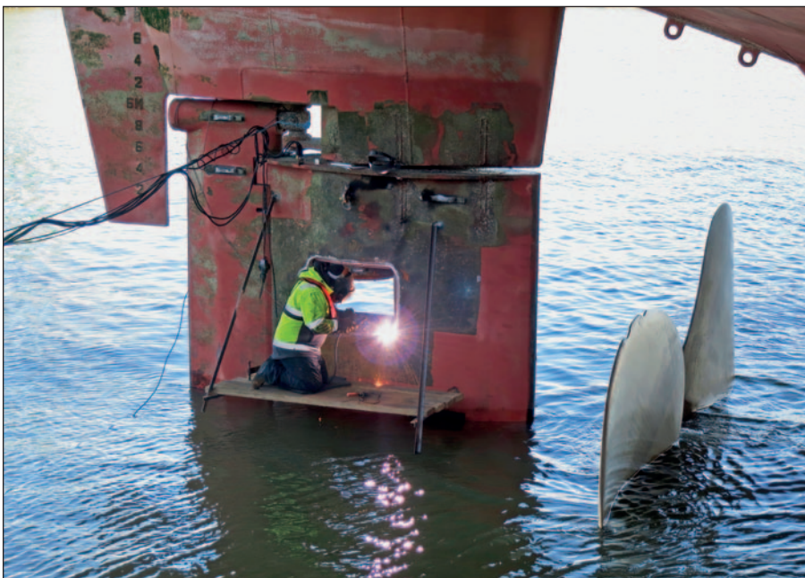
Preparing the rudder for installation of the new cover plates.
