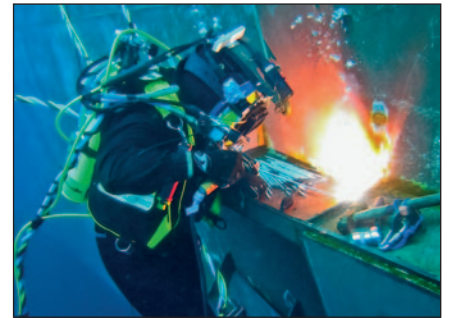
Complex steel repairs carried out afloat 4-9
