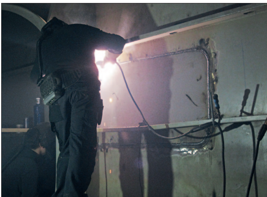
The insert on the ferry was welded by our certified welders.
