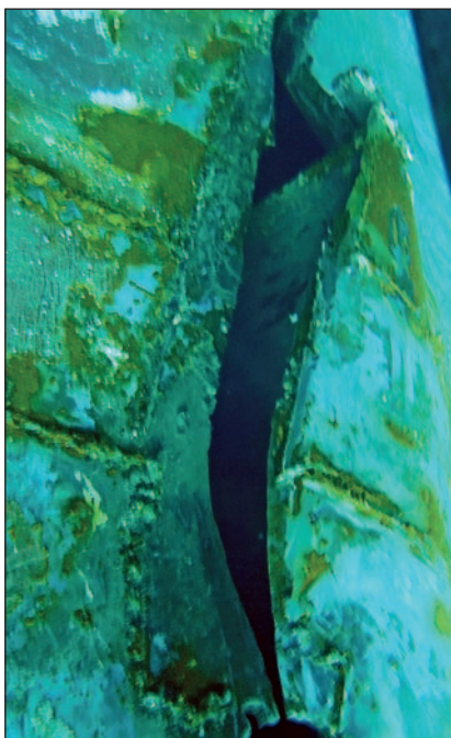
A crack of 1.5 meter appeared after the grounding of a 300-meter bulker, making it impossible for the vessel to continue its voyage.
