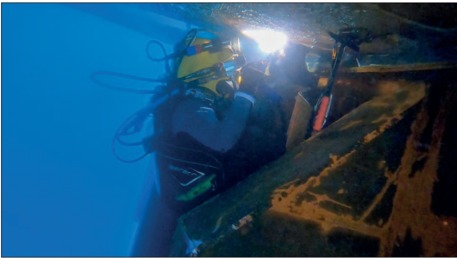
Welding the cofferdam in place.
