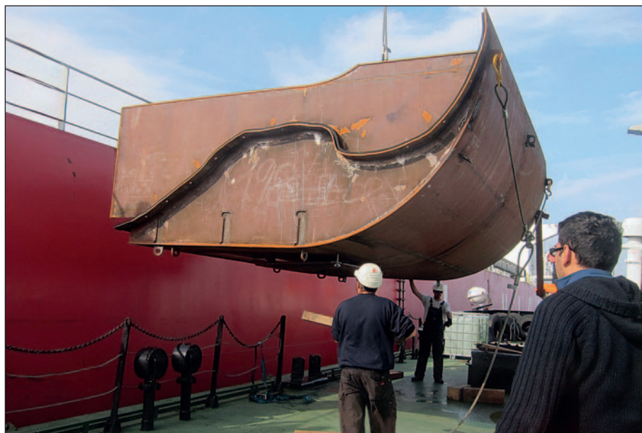
The finished section being lowered into the water in Denmark.
