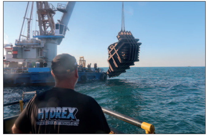
Crane barge moving the 45-ton cofferdam into position.
