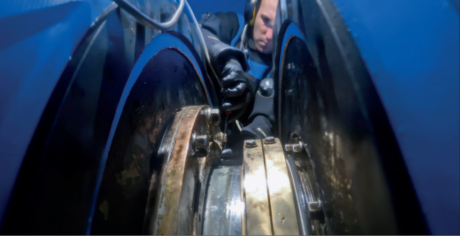
One of our diver/technicians working inside our flexible mobdock in Australia.
