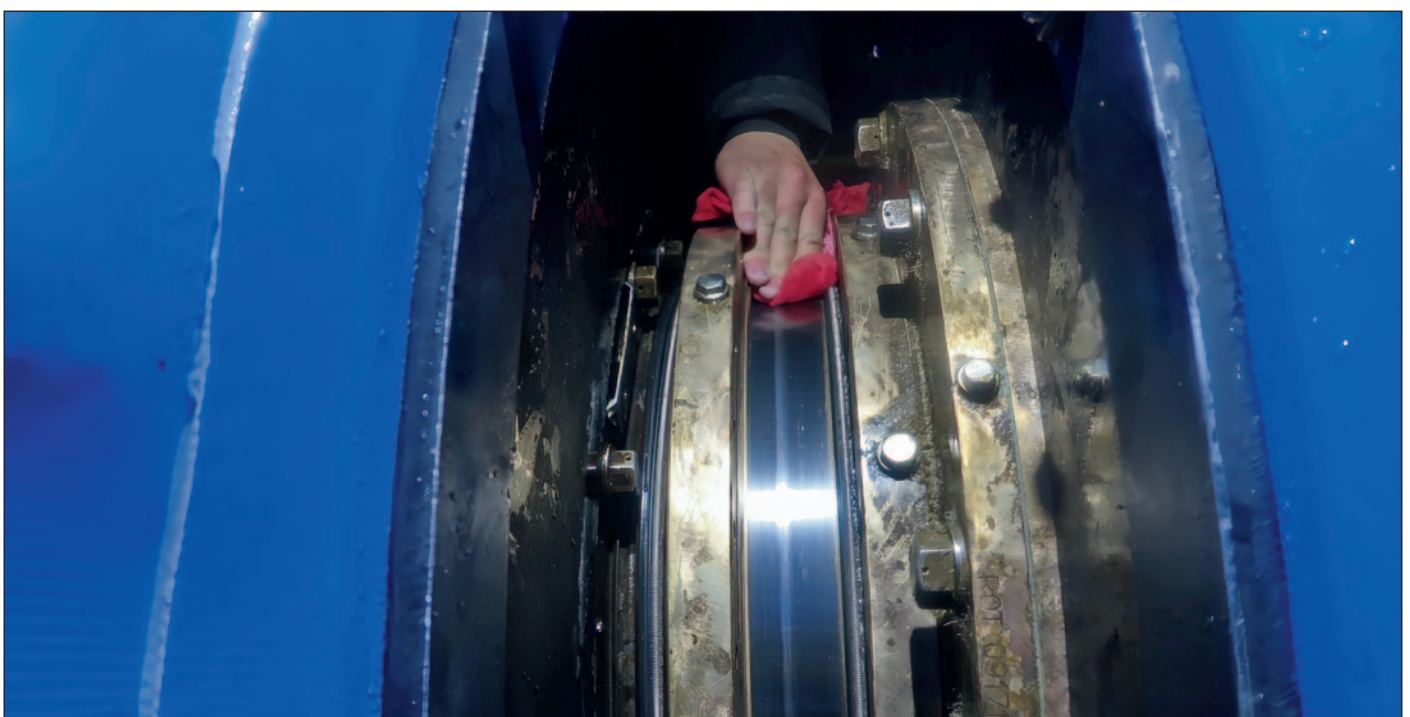
Cleaning the assembly prior to the seal replacement.
