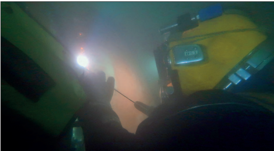
Welding work on the rope guard.
