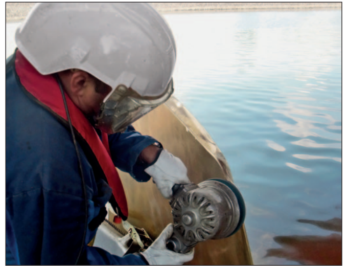
The cropped blades were polished to achieve the best possible efficiency.
