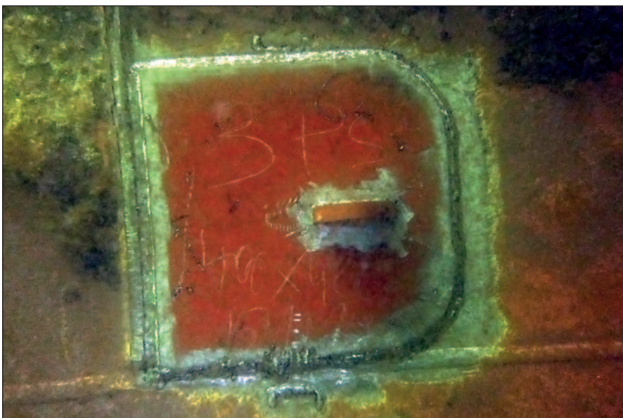
One of six doubler plates installed in Dakar.
