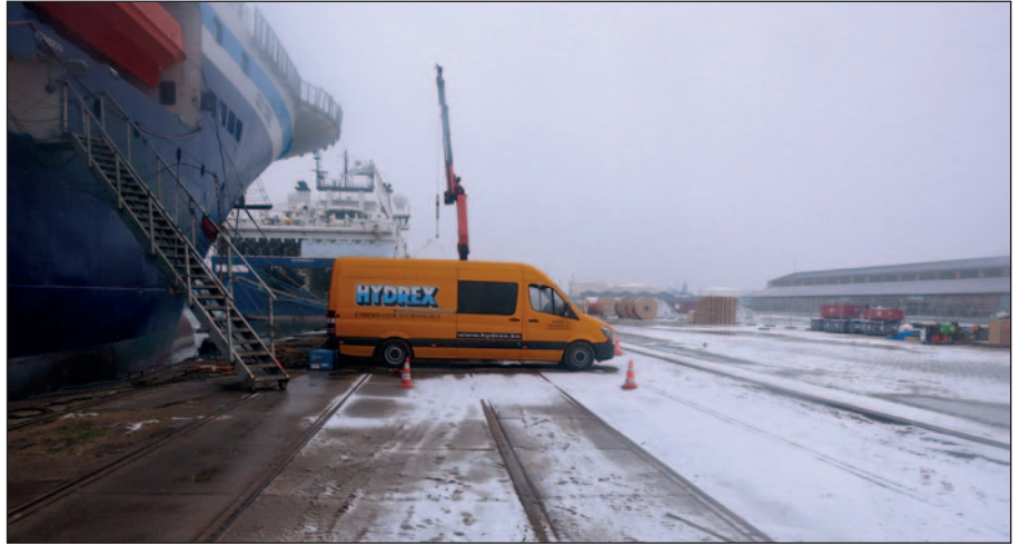
Hydrex team working in winter conditions.
