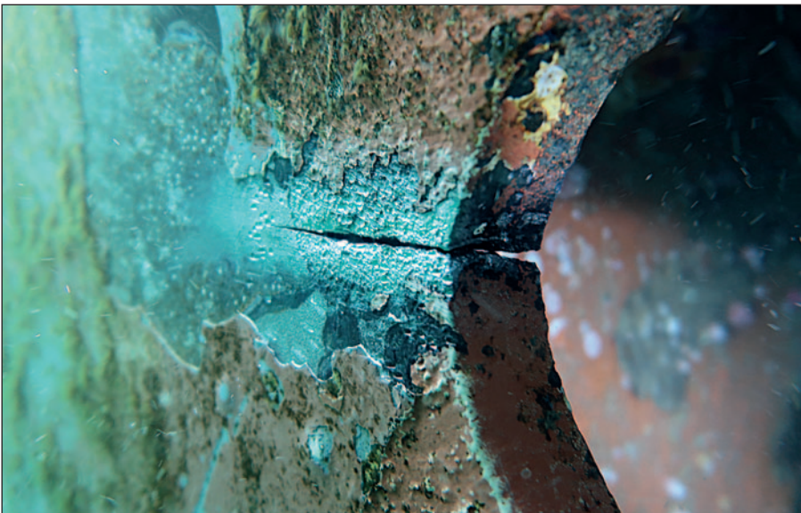
Crack on rudder of bulker in Le Havre.
