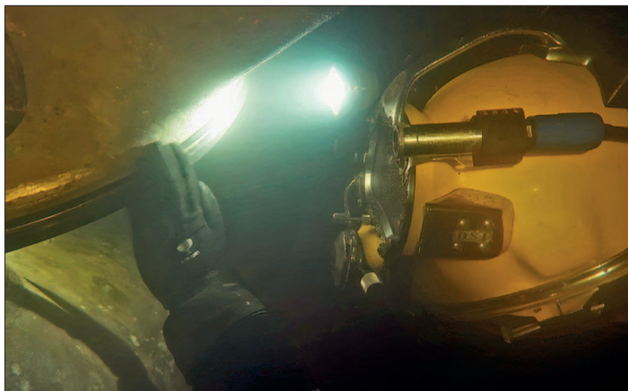
Hydrex diver guiding the new blade into position.
