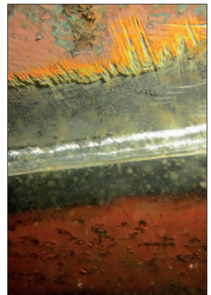
Our divers are all certified welders.
