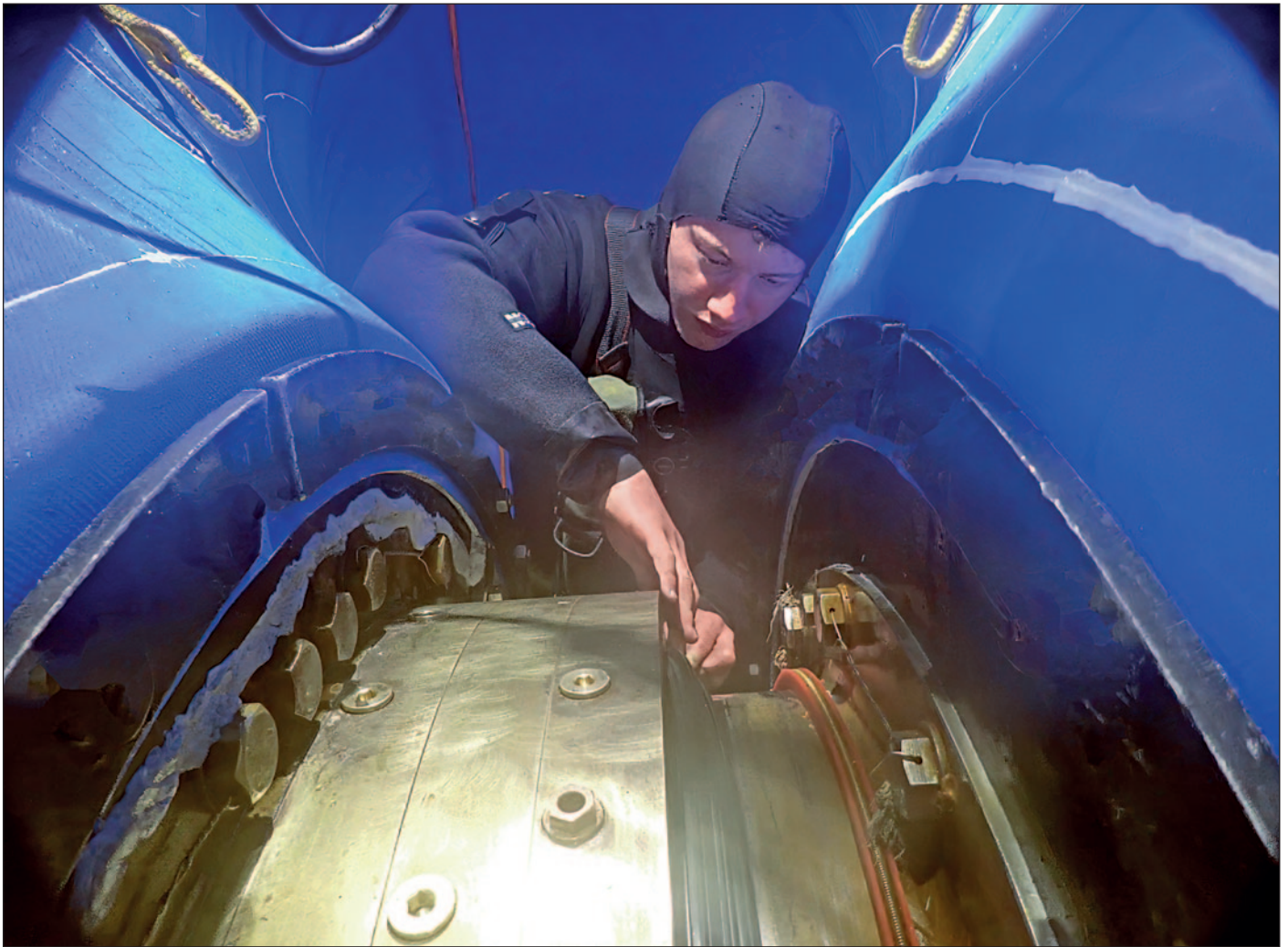
Positioning one of the new seals.
