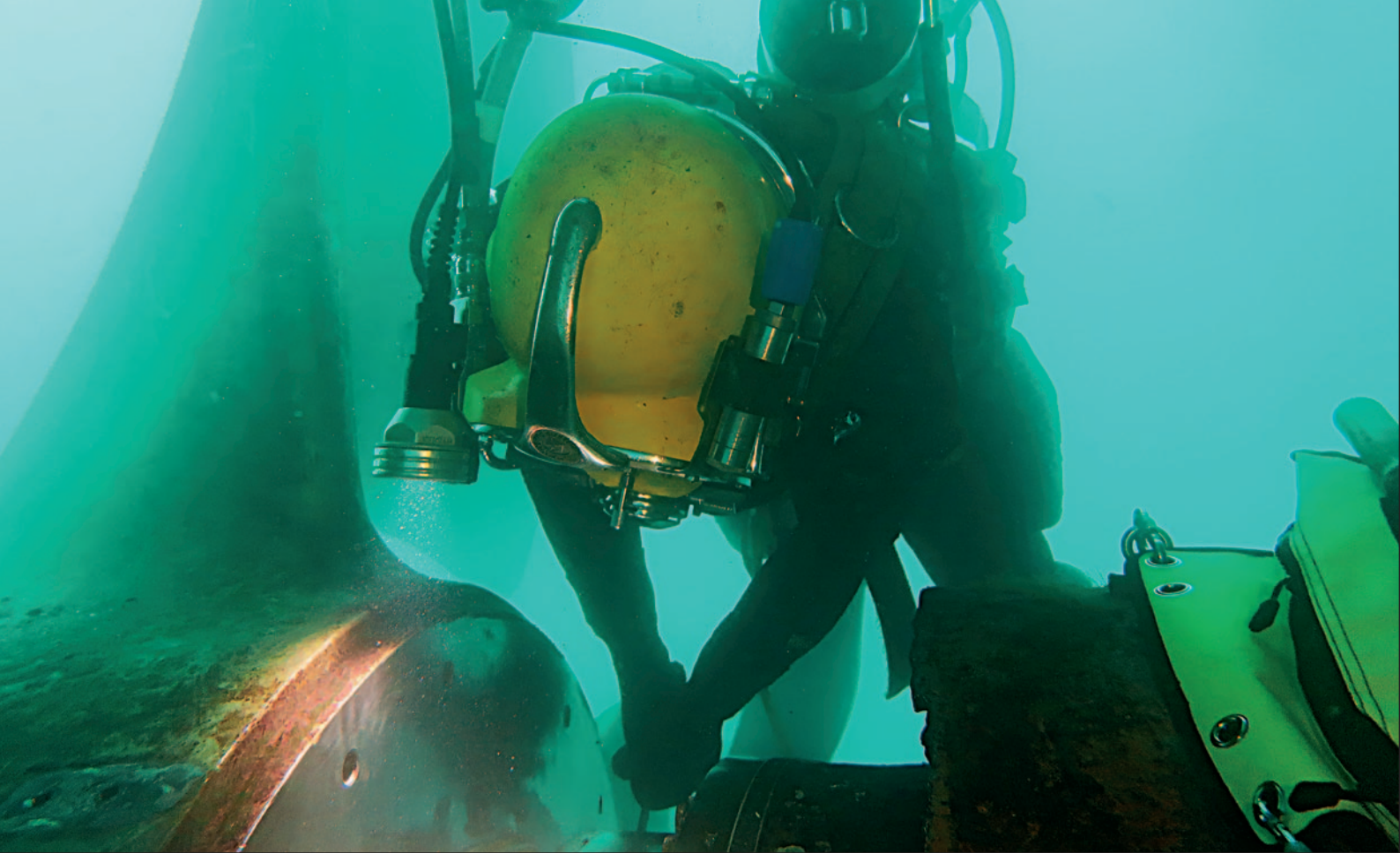
Hydrex diver preparing the assembly for installation of the mobdock.
