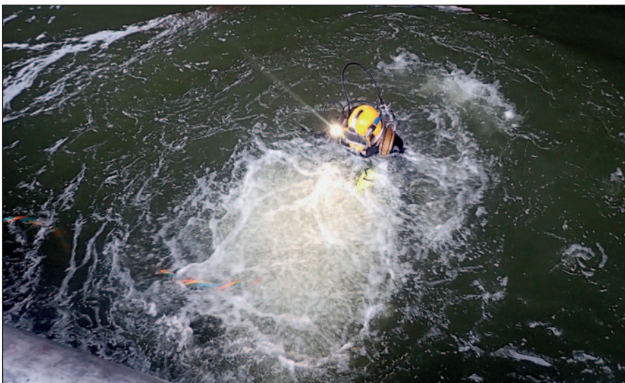
Diver resurfacing after working inside the mobdock.
