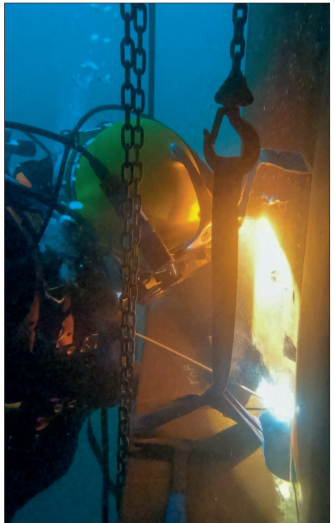
Hydrex diver/welder securing a stiffener.
