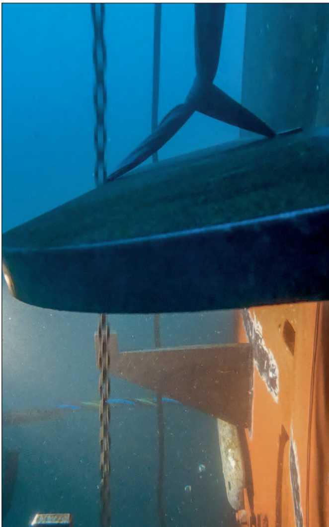
Lowering one of the stiffeners into position.
