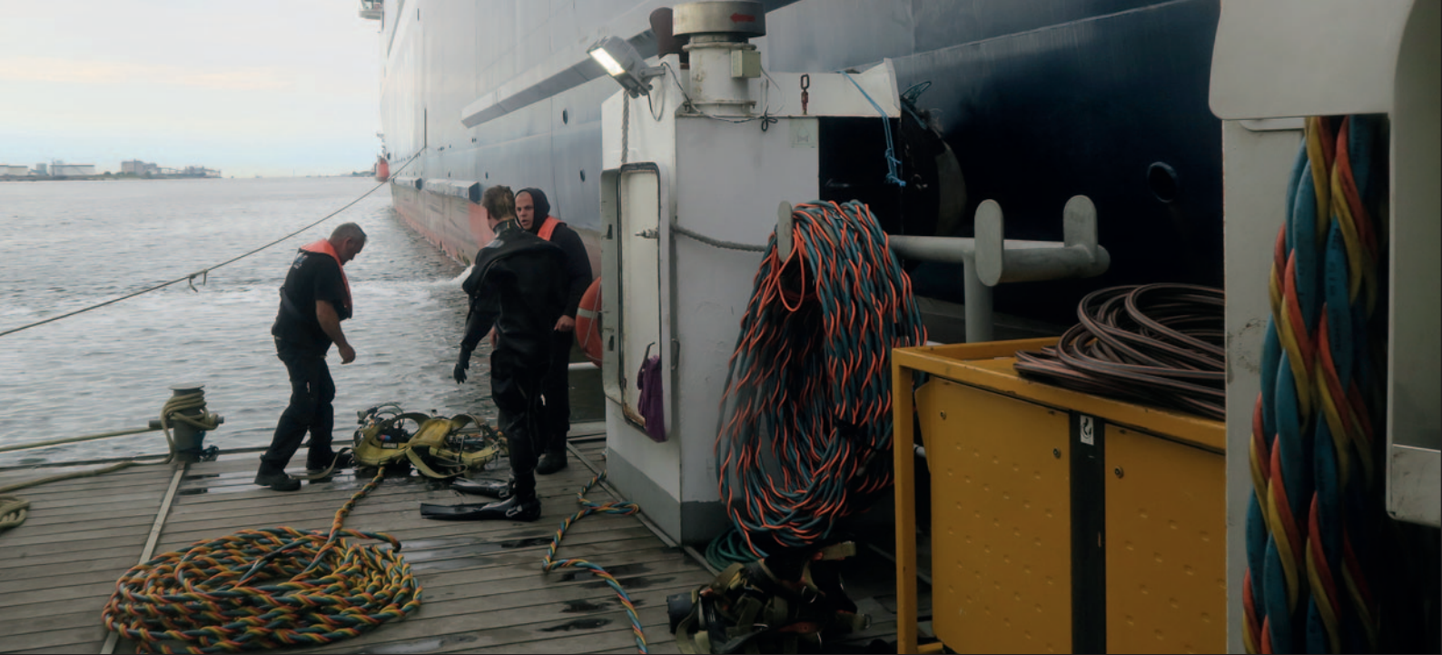
Hydrex work and dive support boat alongside container ship in Rotterdam.
