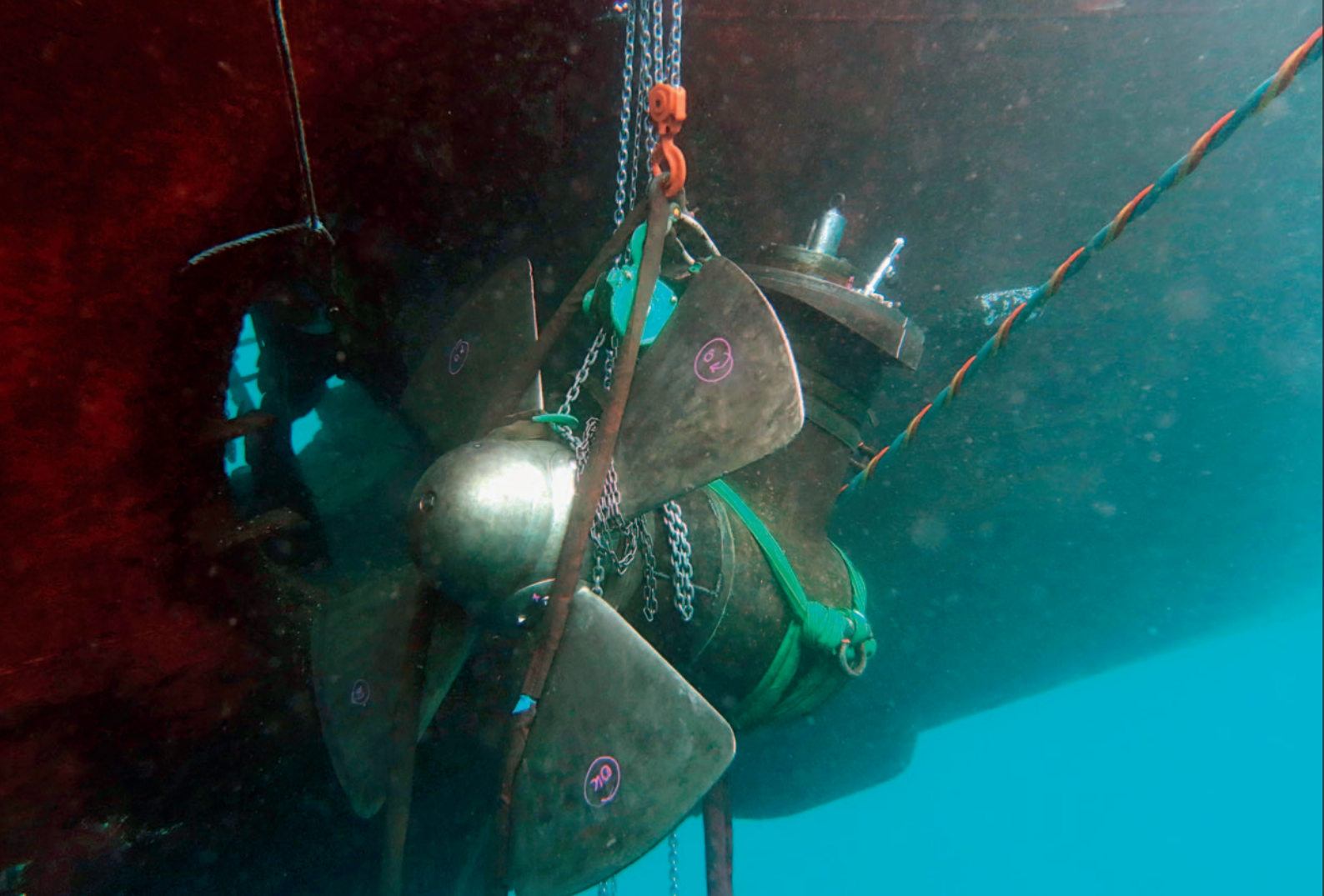
Unit being guided into the thruster tunnel.
