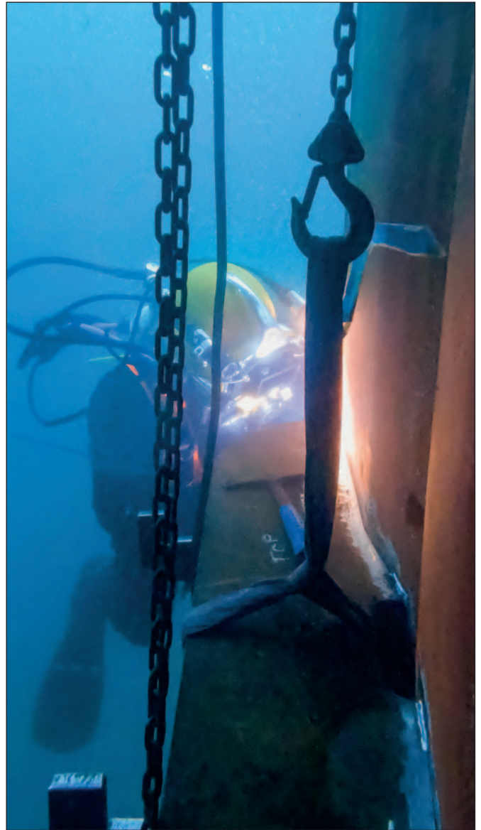
All welding work was carried out by our certified welders.
