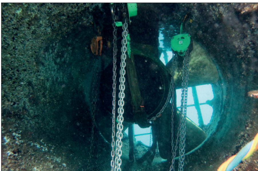
The overhauled unit after being secured.
