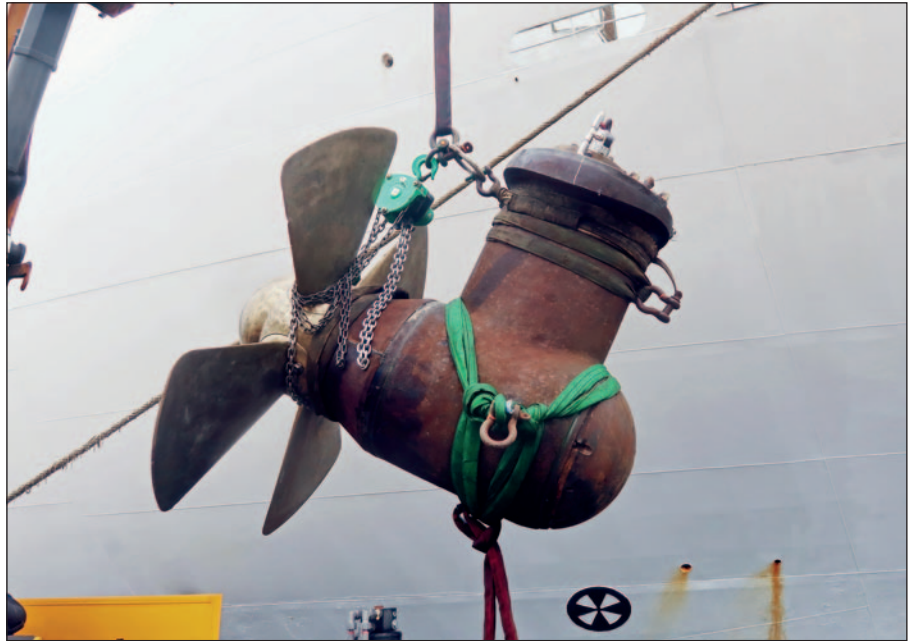
Overhauled thruster unit ready for reinstallation.
