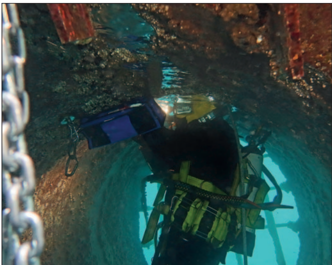
Hydrex diver/technician preparing the tunnel for reinstallation of the thruster.
