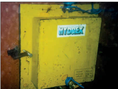
Cofferdam placed over crack.
