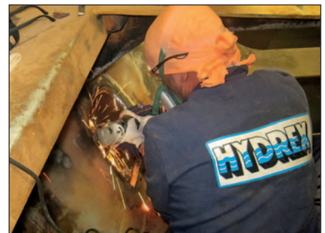
Preparing the edge of the opening for the new insert.
