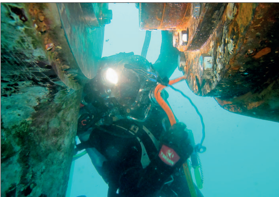
Inspection of the seal assembly prior to installation of flexible mobdock.
