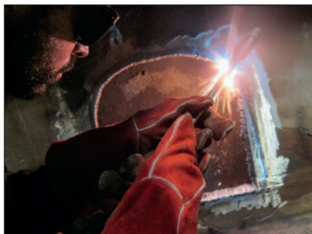
Removing the damaged area.
