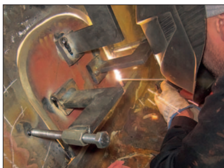
Insert tacked in place.
