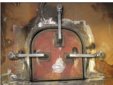
Insert cut and fitted.
