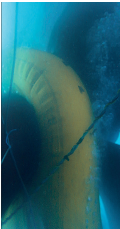
Our flexible mobdock allows for underwater work on the seal assembly.
