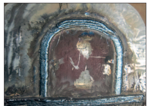
Full penetration weld.
