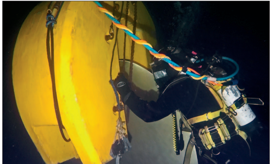
Hydrex diver positioning cold-straightening machine.
