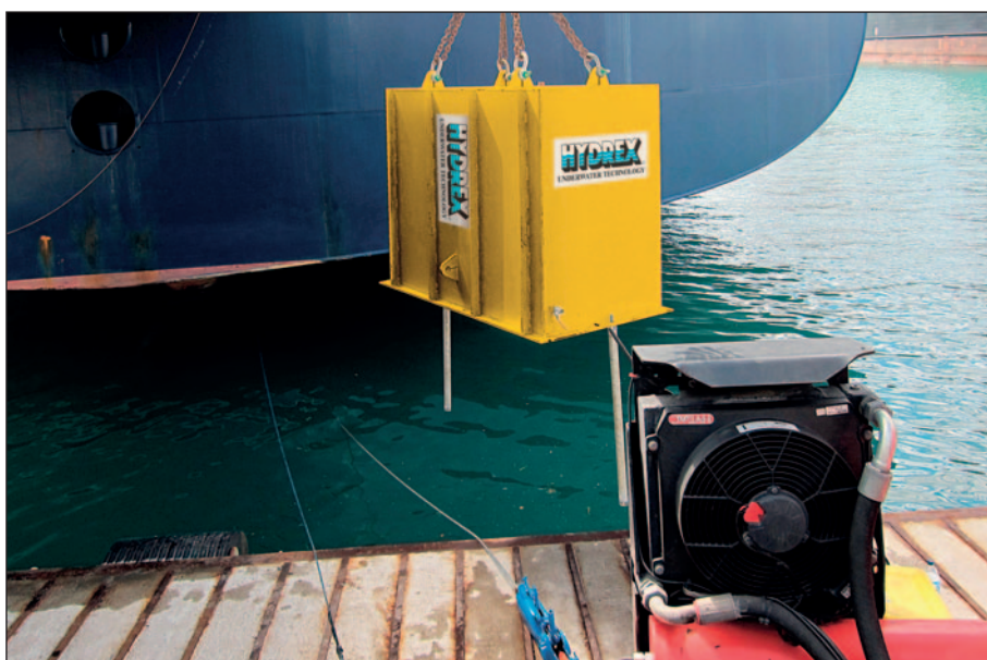
A special cofferdam was constructed to replace spinner cone bolts without going to drydock.
