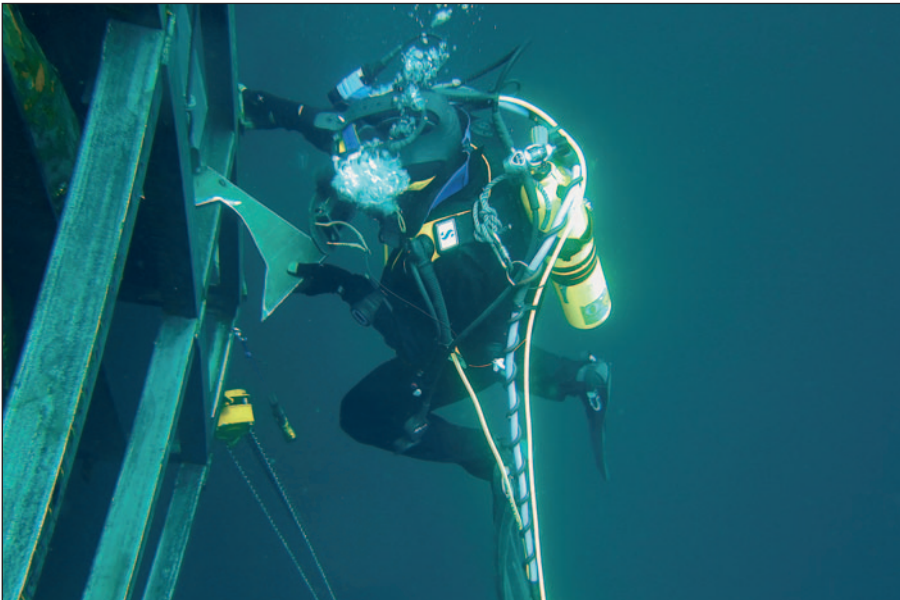
Special cofferdam designed to cover a 1.5 meter crack.
