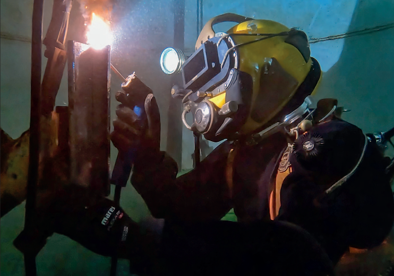
Underwater welding practice in the dive tank makes it easier for our teams to operate on the job.
