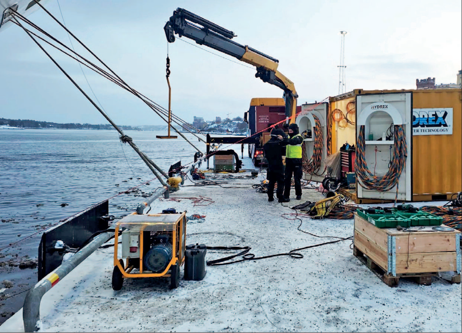
Hydrex diving station and equipment next to ferry in Stockholm.
