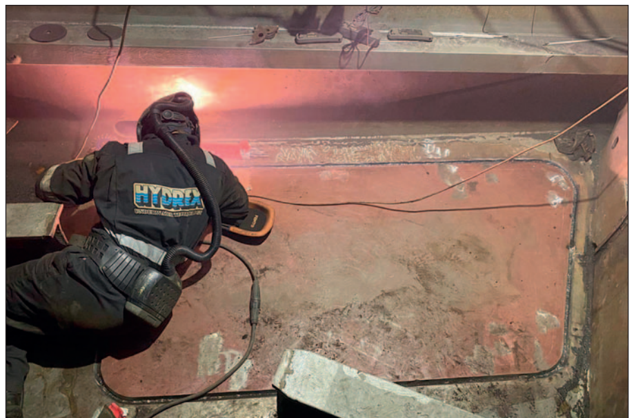
Hydrex diver/welder welding one of the inserts in Dakar.
