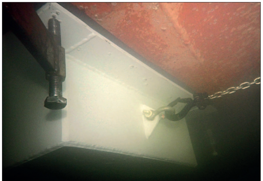
A cofferdam was installed on the hull, covering the damaged area.
