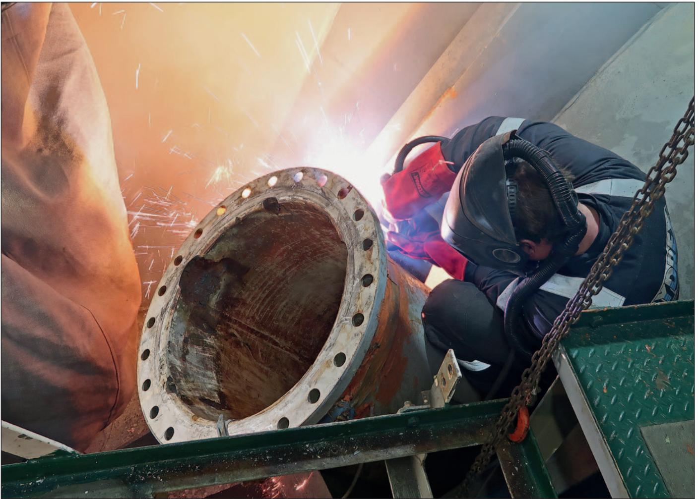
Hydrex technician cutting away the old pipe.
