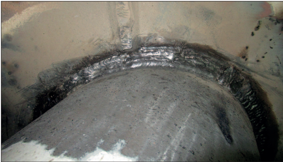
New scrubber pipe after welding.
