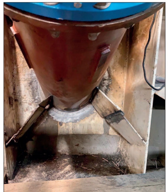
All welding work is done following our class approved procedures.
