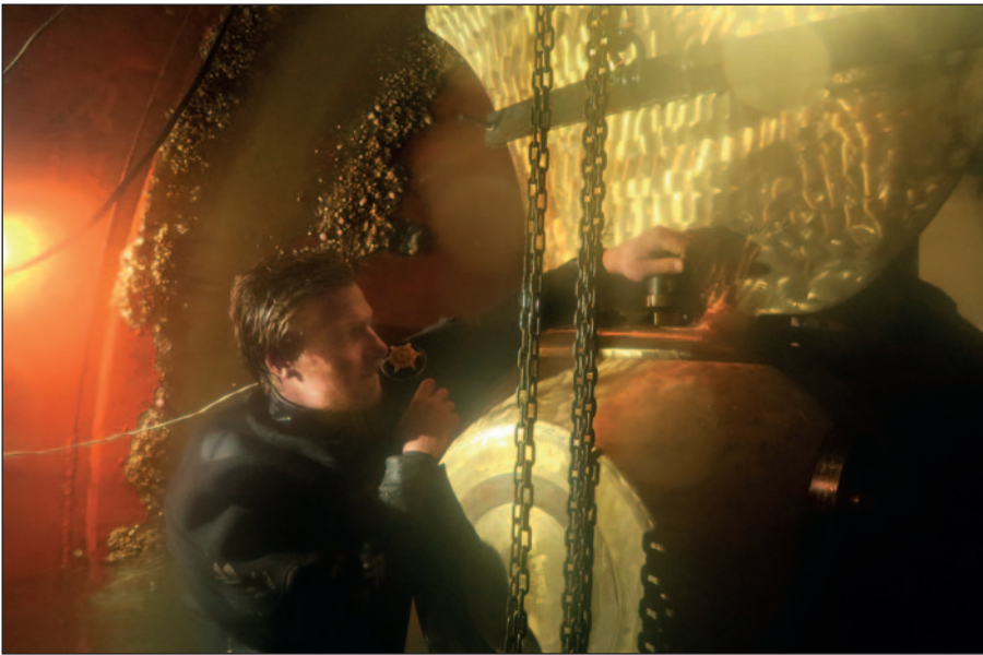
Installing one of the blade bolts in Italy.
