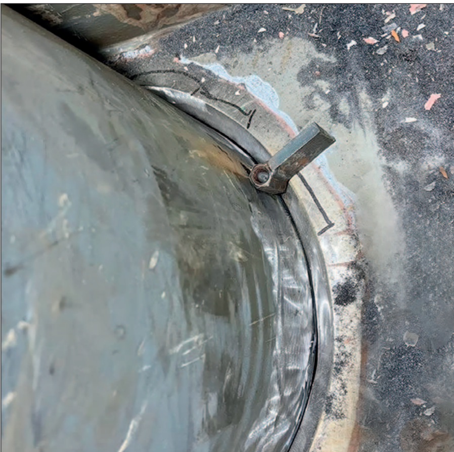
Scrubber pipe secured and ready for full penetration weld.
