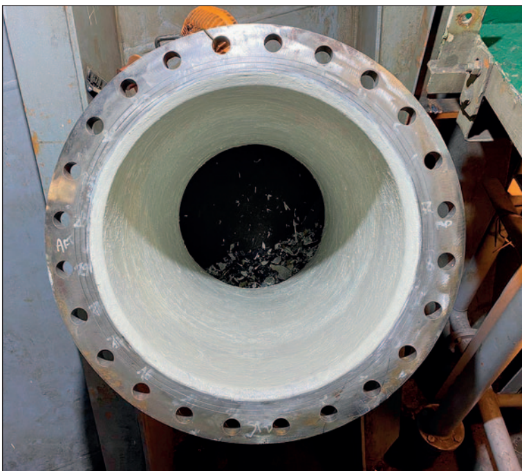
New scrubber pipe coated with Ecoshield.
