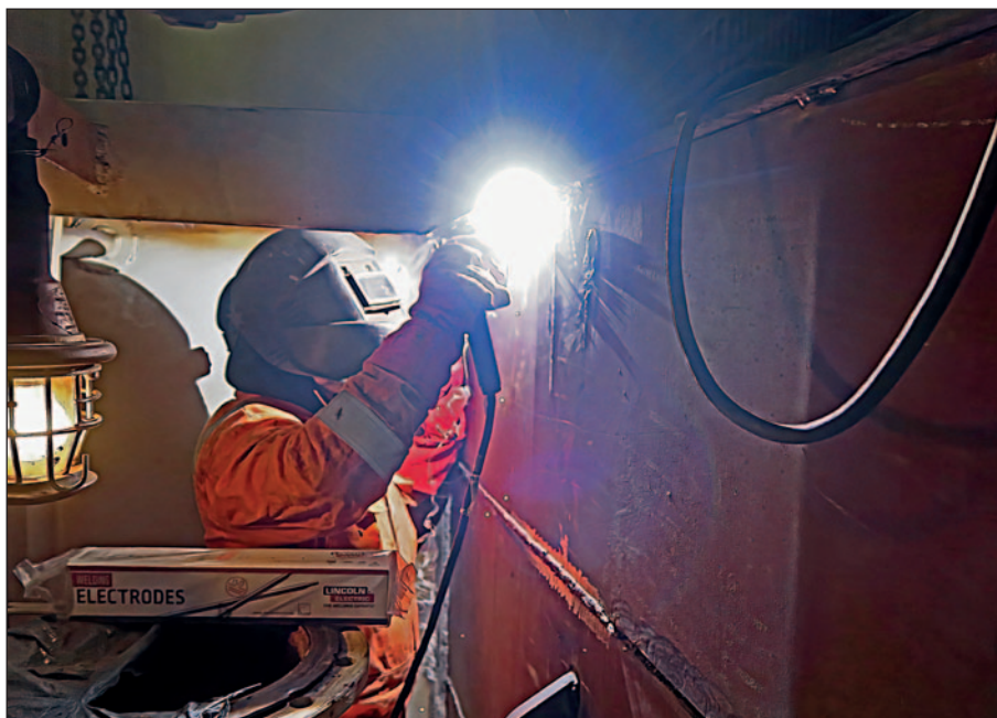
Securing new inserts in Rotterdam with full penetration weld.
