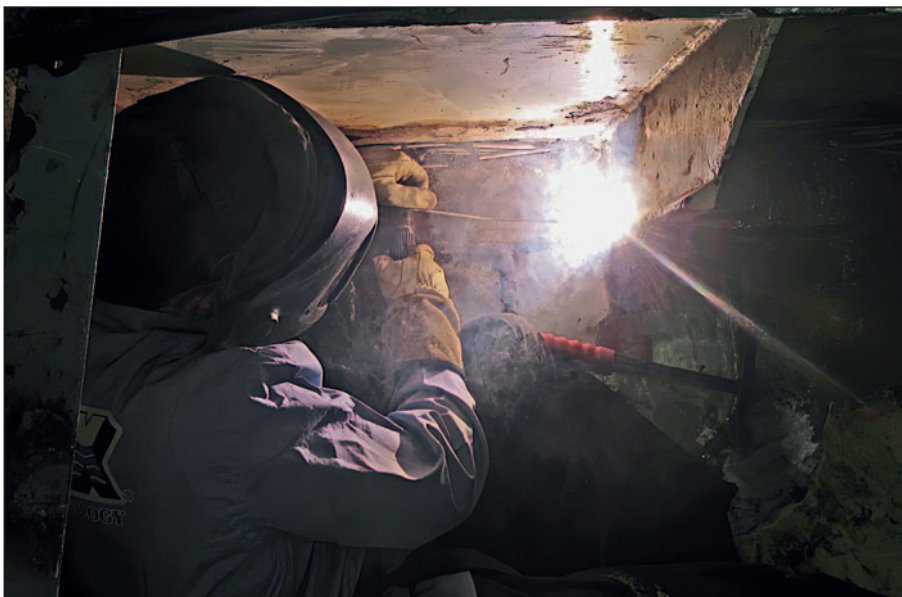
Hydrex welder during operation in Amsterdam.
