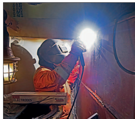
Permanent shell plating repairs without drydocking 4-8
