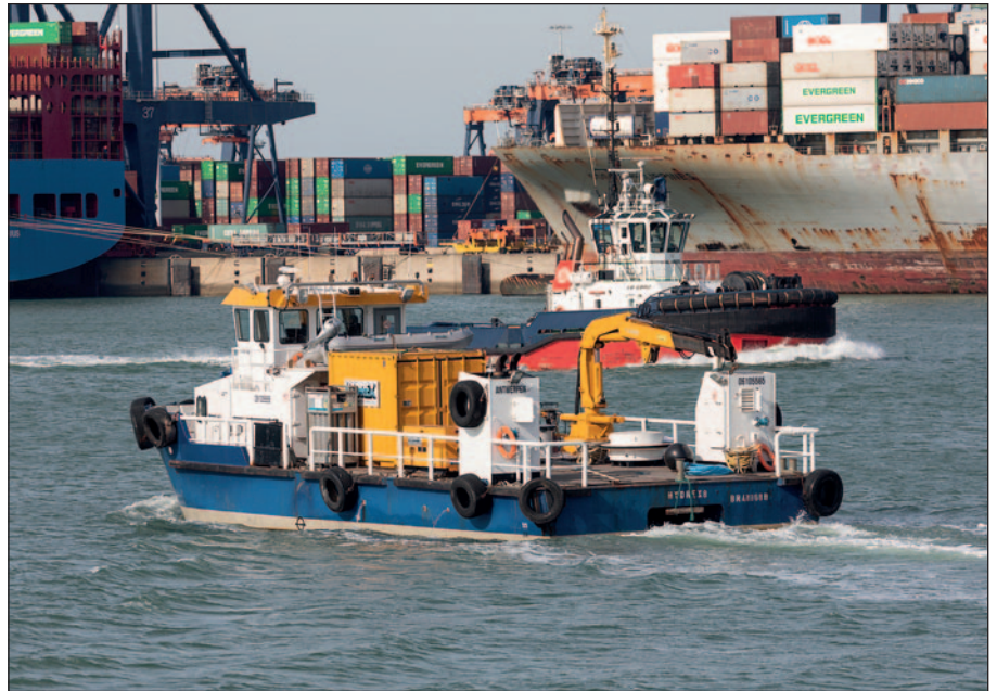
Hydrex workboat on its way to a repair site in Rotterdam.
