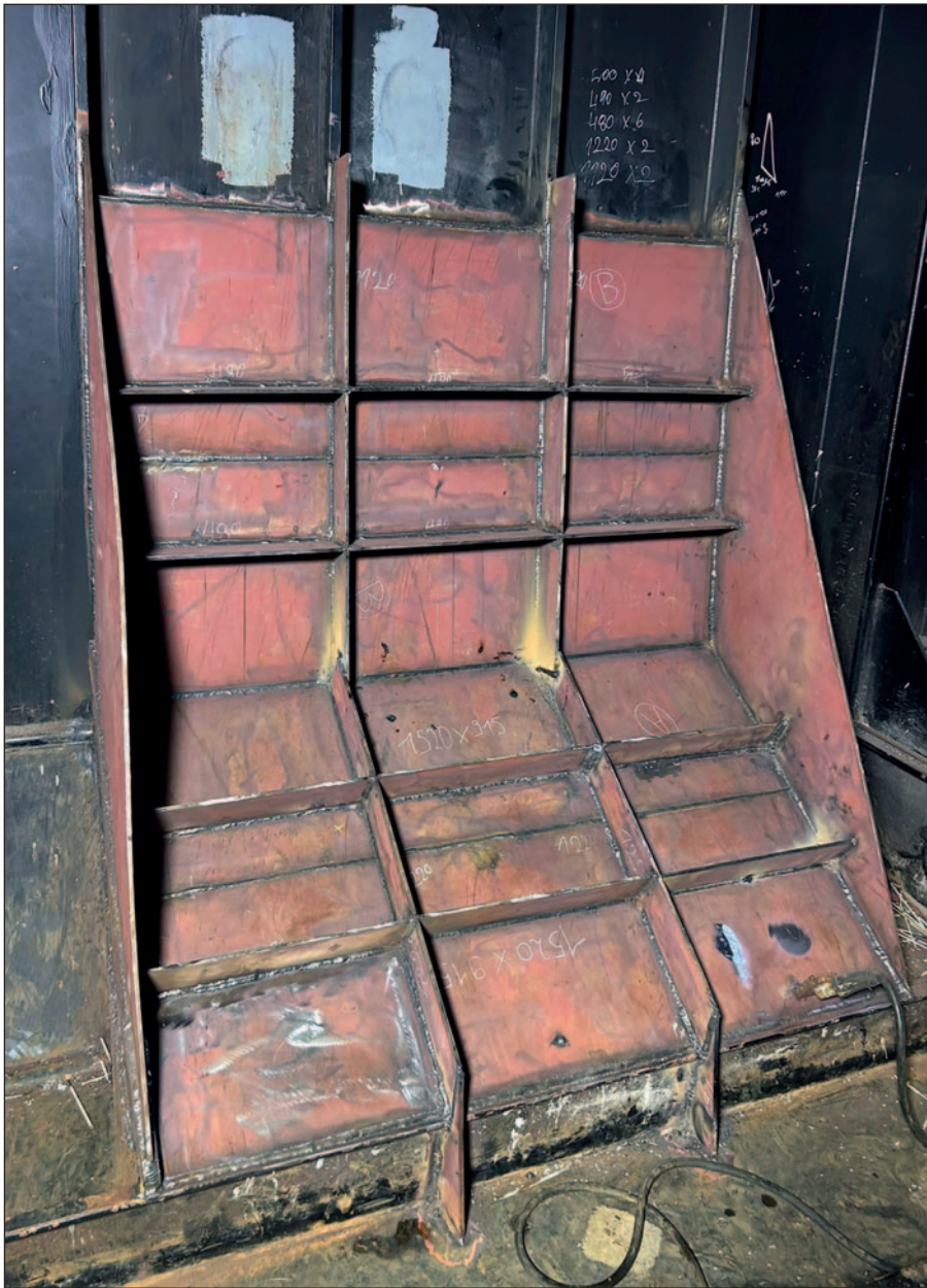
Cofferdam ready and approved by the independent inspector.
