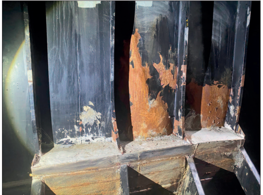
Concrete box installed over the damaged area by the crew.
