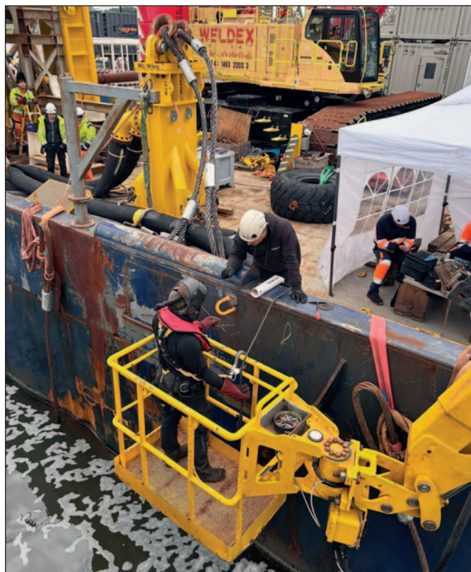
During the operation our team performed some small additional work for the customer, like installing new pad-eyes on the side of the hull.
