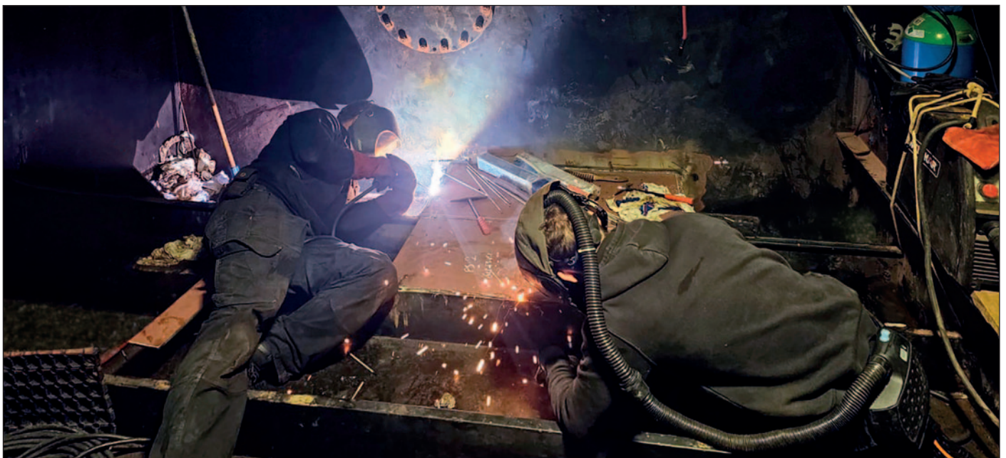
Hydrex welders working on one of the cofferdams in void tank 6.
