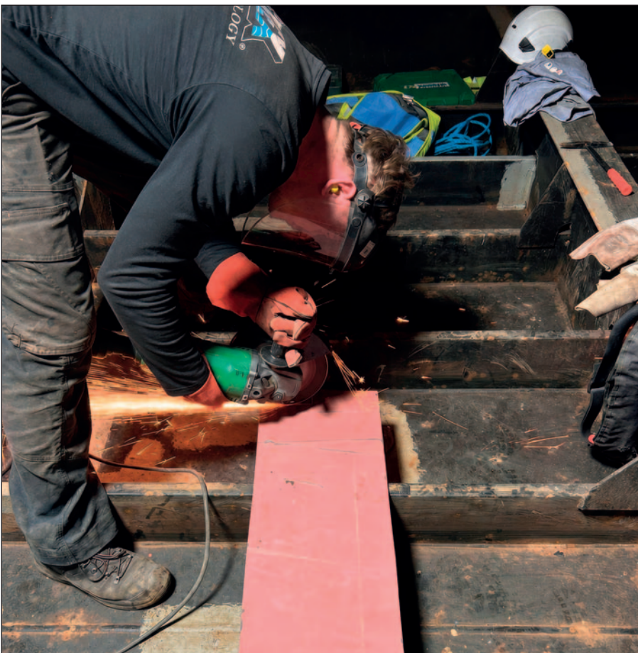
Cutting a section of one of the three cofferdams.
