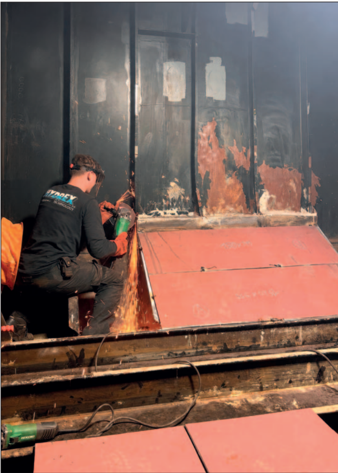
Cutting work on the edges of the cofferdam in void tank 4.
