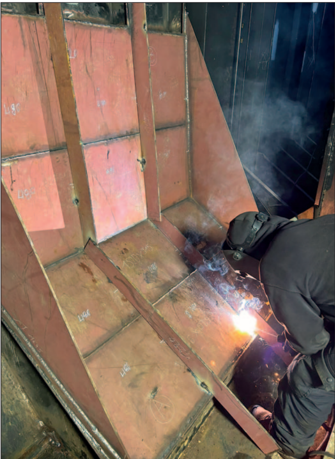
The cofferdam was constructed in sections, following the shape of the hull.
