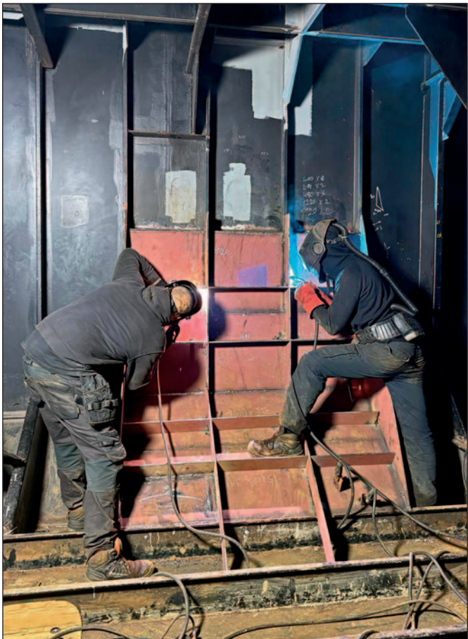
Hydrex certified welders installing steel frames to reinforce the cofferdam.
