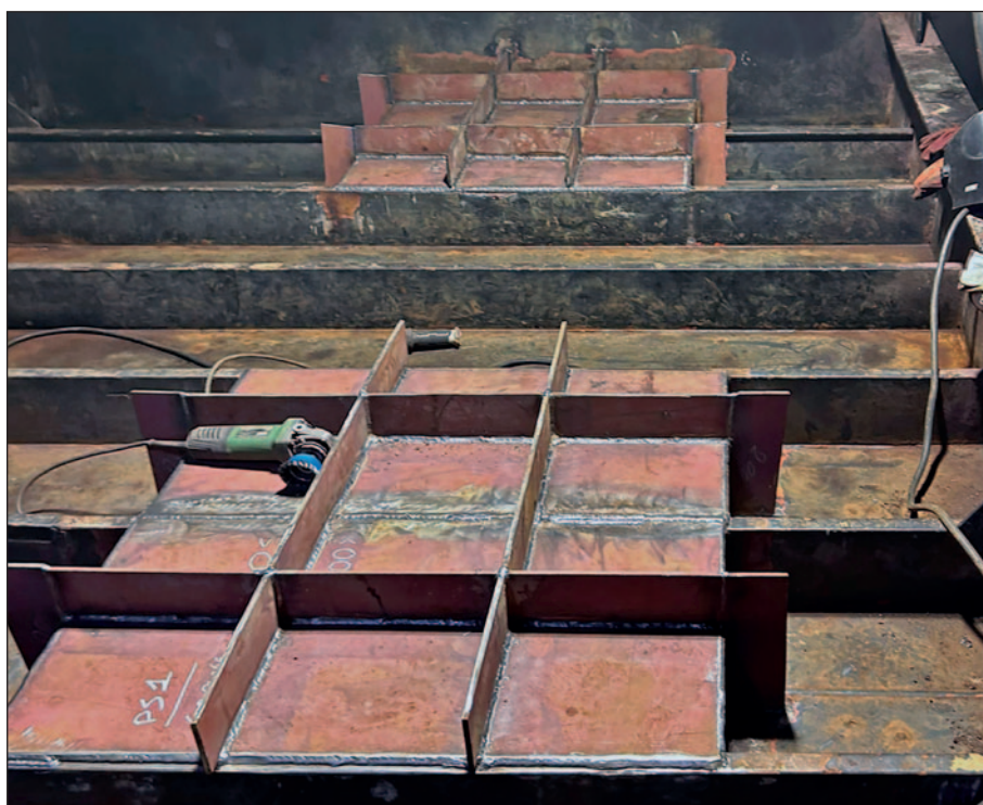
Two cofferdams were installed in the void tank 6.
