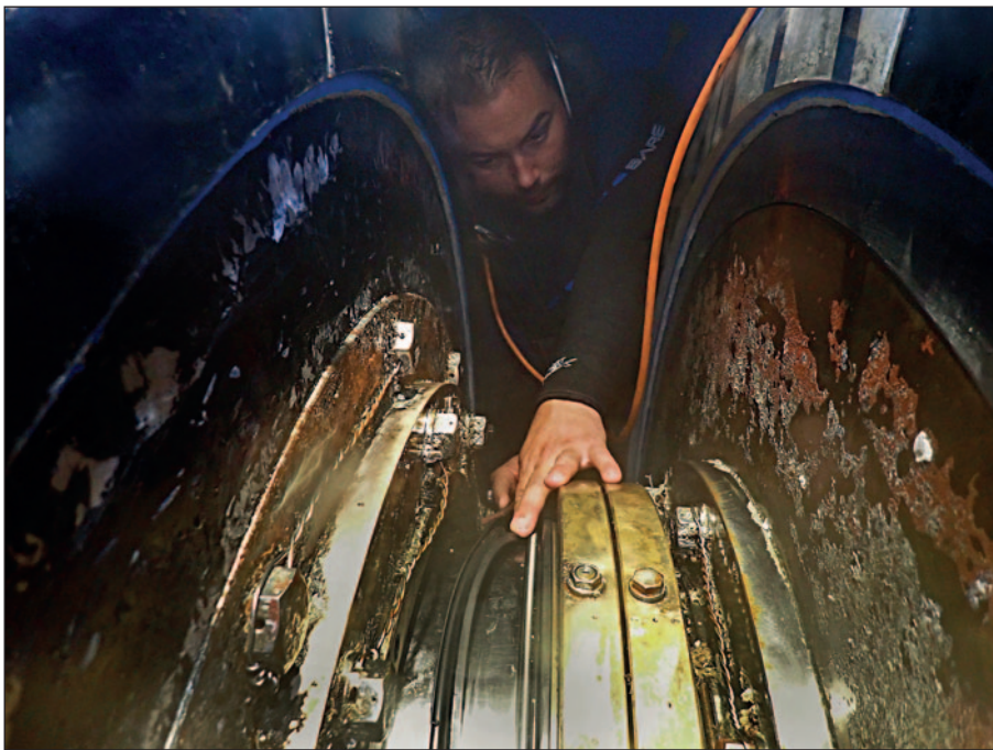
Diver working on the seals inside flexible mobdock.
