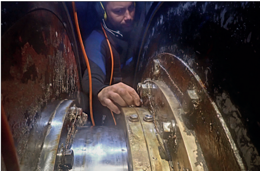
Reinstallation of the assembly after seal replacement.
