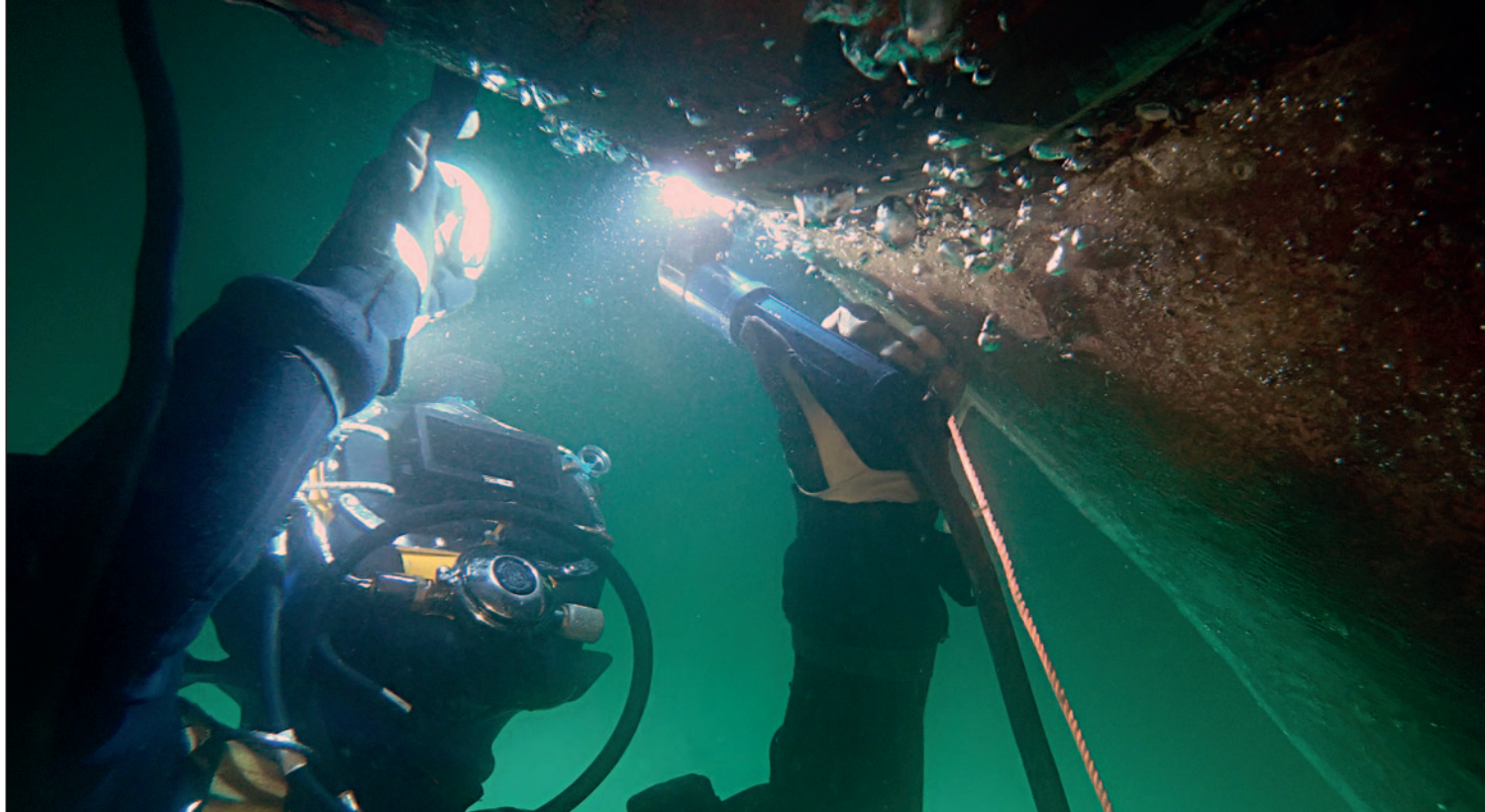
Reinstalling the ropeguard to finalize the operation.
