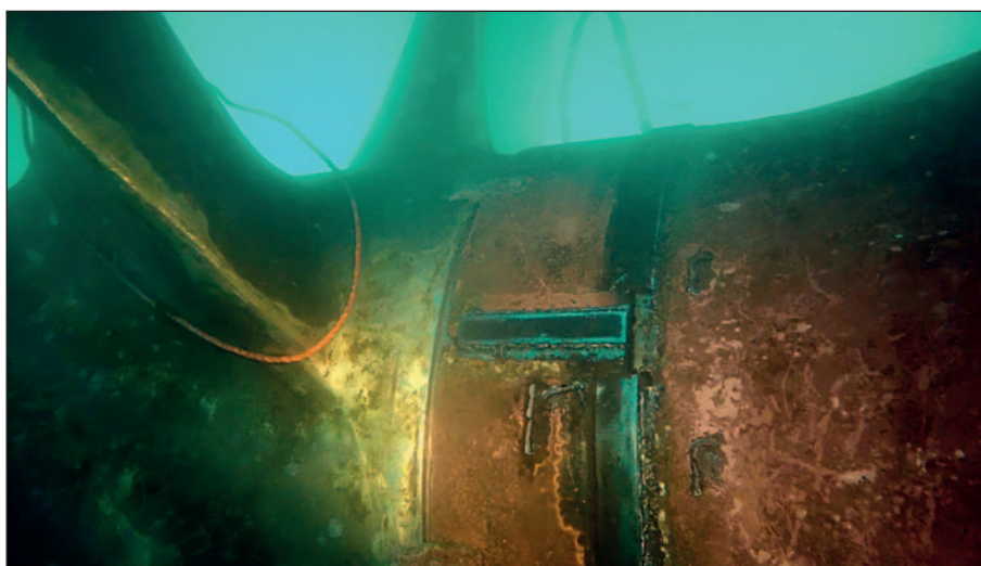
The stern tube seal assembly with ropeguard after conclusion of the repair.
