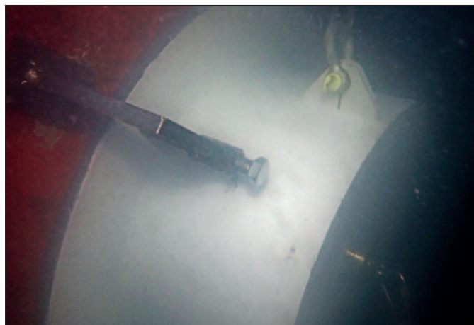
Cofferdam installed on cruise ship in Panama.
