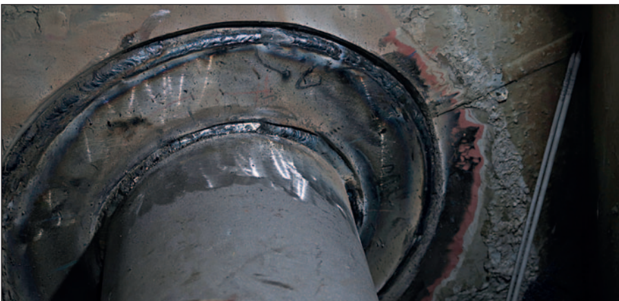
New pipe and surrounding shell plating on bulk carrier.
