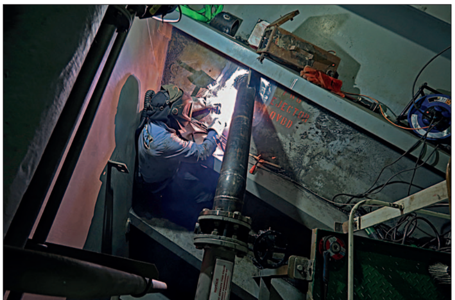
Reinstallation of the new pipe in Rotterdam.
