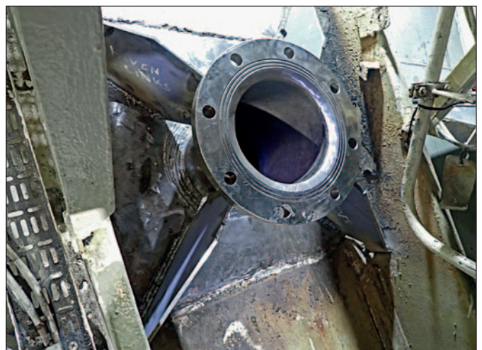
New overboard pipe after reinstallation of the brackets.
