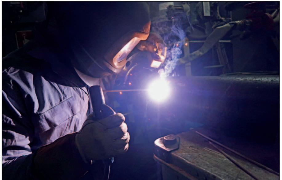
Hydrex certified welder preparing the new discharge pipe for installation.
