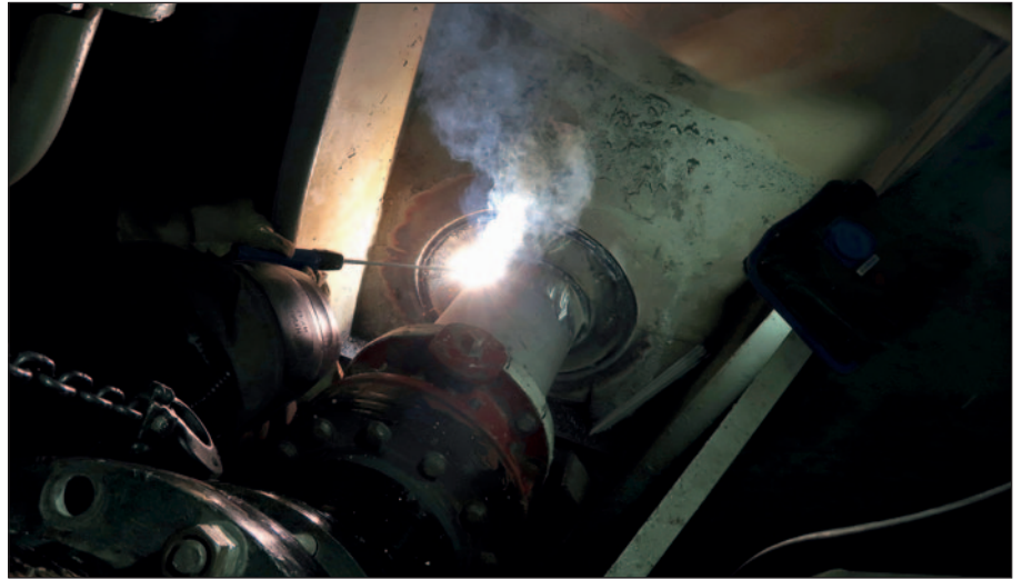
Welding work on overboard pipe in Dunkirk.
