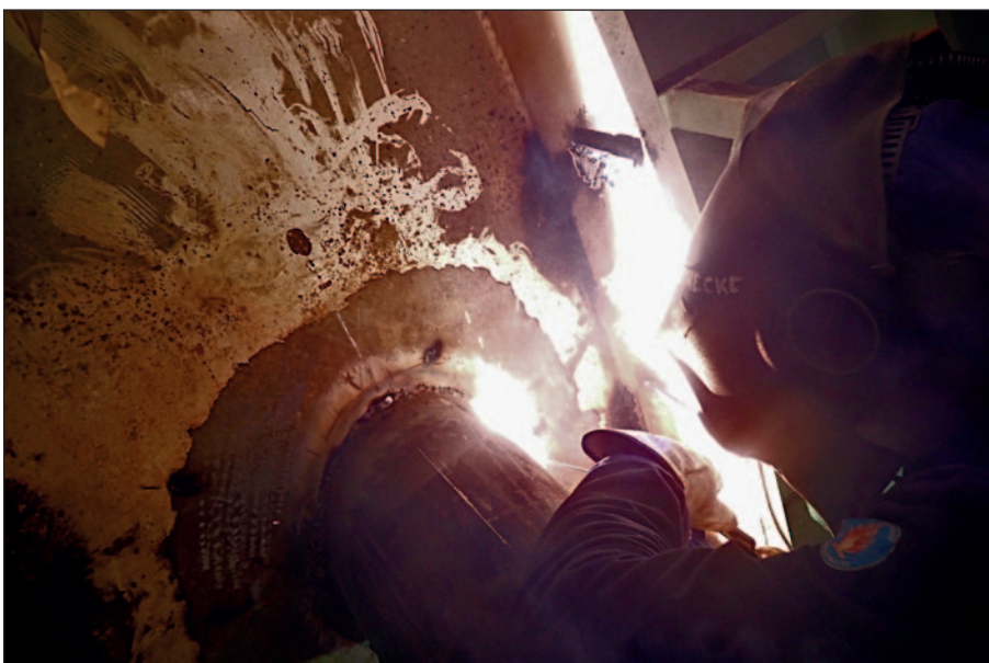
Welding work on new scrubber overboard pipe in Jebel Ali.
