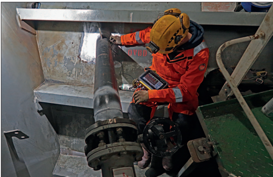
NDT inspection by an independent inspector.
