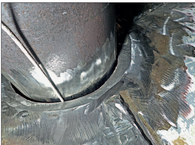
The new pipe positioned and ready to be welded.
