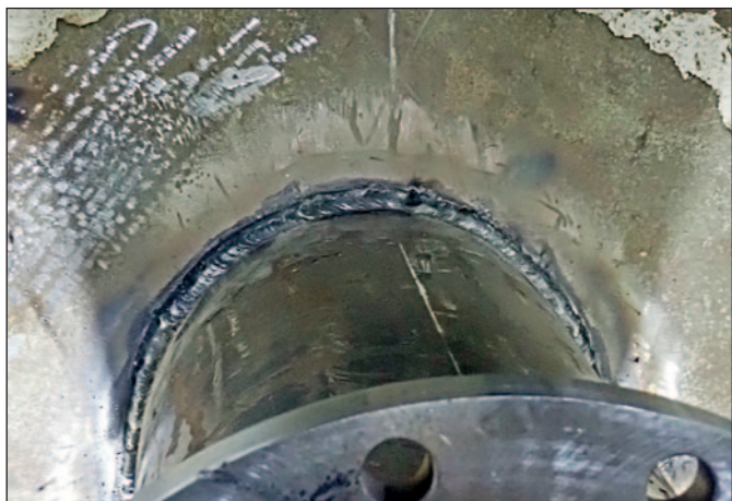
The new pipe on the vehicle carrier was fitted with full penetration welding.
