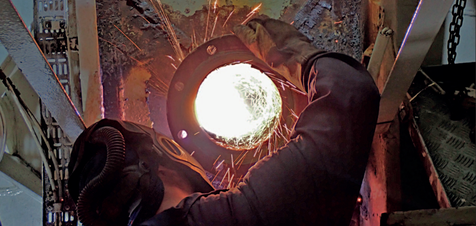
Cutting away the old overboard pipe.
